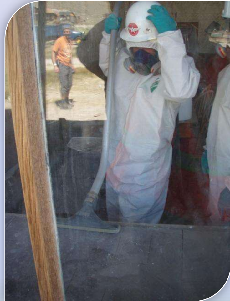
HEPA vacuuming inside Wheaton-Hollis Hotel
