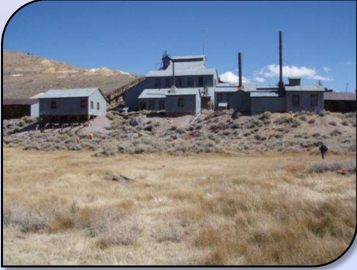
Standard Mill (inside & slope)
