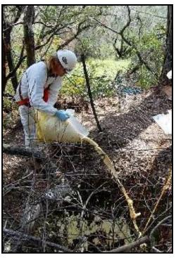
POURING PUF INTO THE SHAFT
