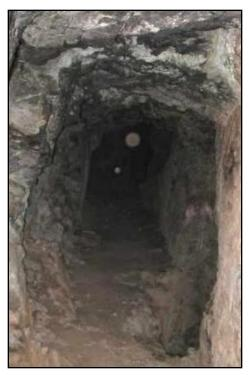
**BEFORE** (Note, there is an extremely hazardous vertical shaft on the right side of the floor of this adit.)
