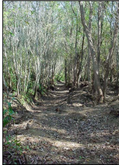
Channel after maintenance work.
