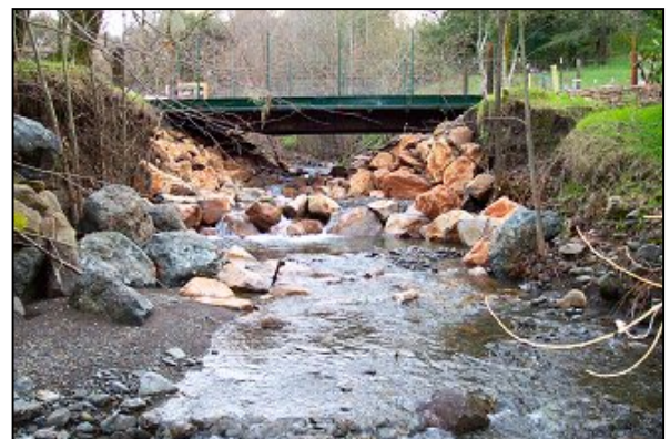
Culverts removed and replaced with free spanning railcar bridge – January 2005.
