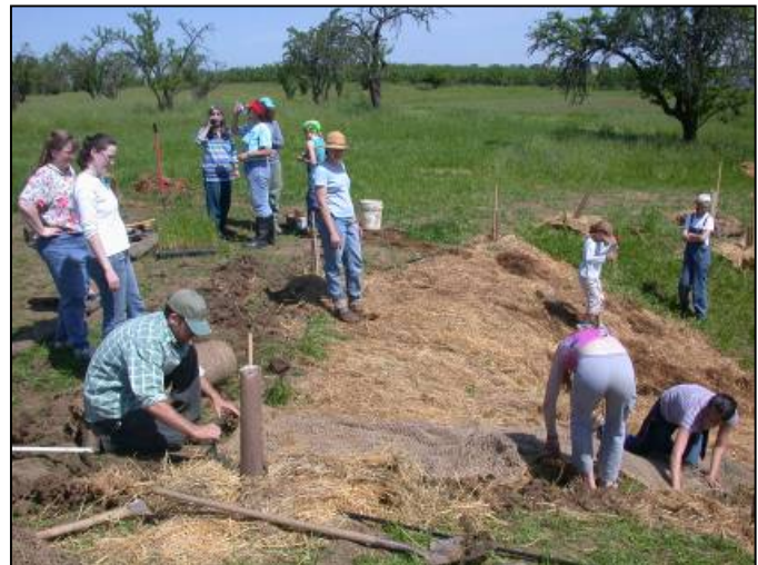
Volunteers in the SLEWS program place netting for gully protection on property along Little Lamb Valley Slough.
