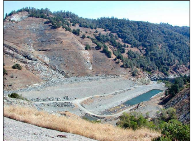
Overview of the Auburn Dam site. The Bureau of Reclamation is finalizing plans to reclaim the area.
