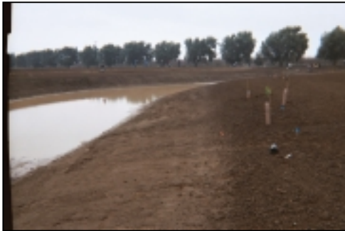
Tailwater pond installation and revegetation project
