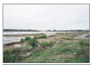
Arroyo Grande Creek control channel breached, partly due to blockage from accumulated sediment.
