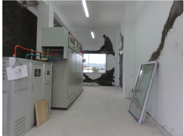
(b) Interior of control building
