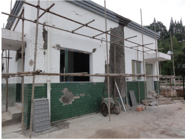
(a) Exterior of control building
