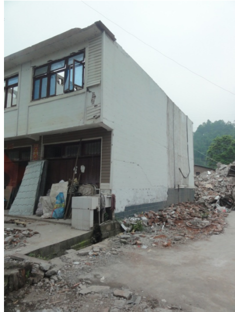
Fig. 11. Damaged building with roof collapse.
