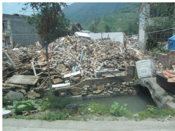
Fig. 9. Debris from collapsed building (Photo by Dr. Craig A. Davis).
