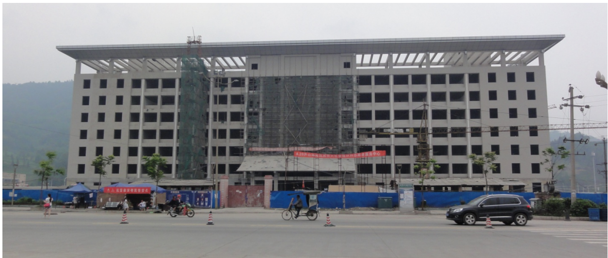
Fig. 14. Government building under construction in New Lushan Town.
