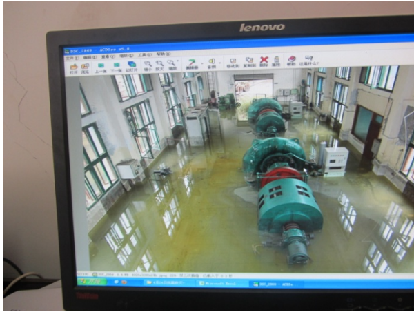
Fig. 23. Hydropower plant made inoperable by flooding. (Photograph by Dr. Craig A. Davis)
