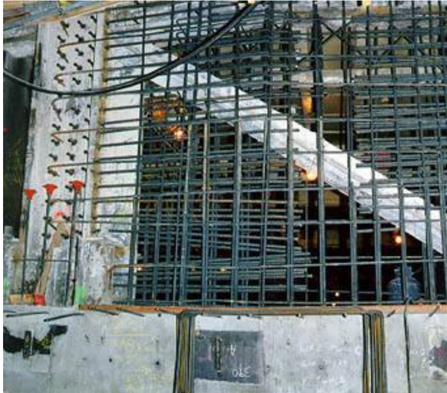
Figure 12: Rebar for new concrete shear wall at basement level
