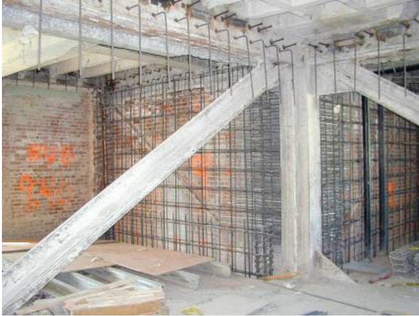
Figure 13: Rebar for new concrete shear wall in tower
