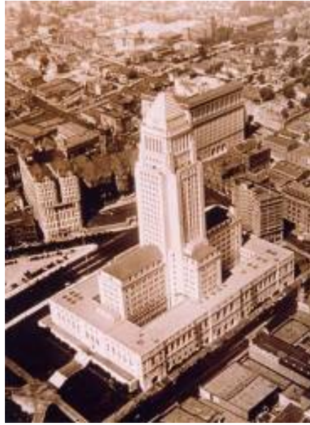
Figure 1: Aerial view of building
