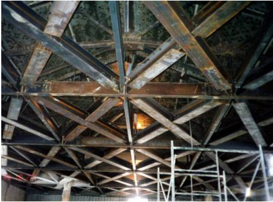
Figure 15: New horizontal steel truss diaphragm at 11 th floor
