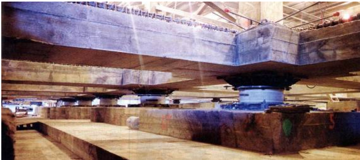
Figure 14: New basement diaphragm in construction
