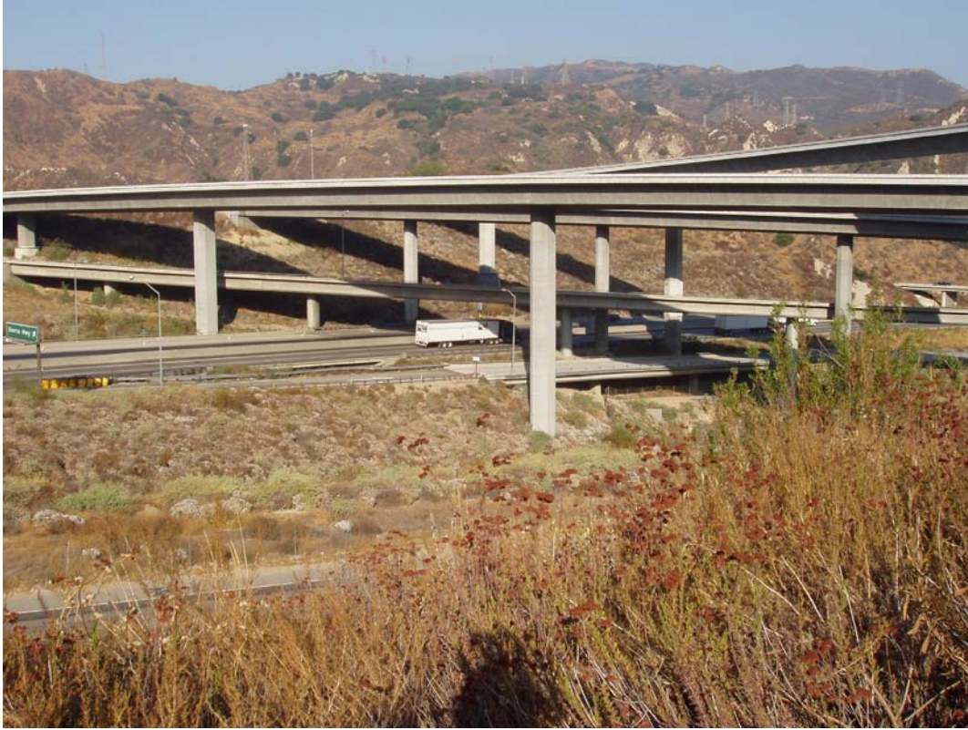
Figure 3. North Connector, looking east.
