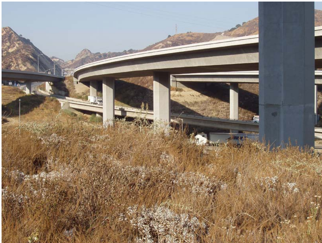
Figure 2. North Connector, looking northeast at Abutment 11
