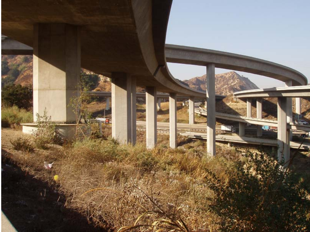
Figure 1. North Connector, looking north
