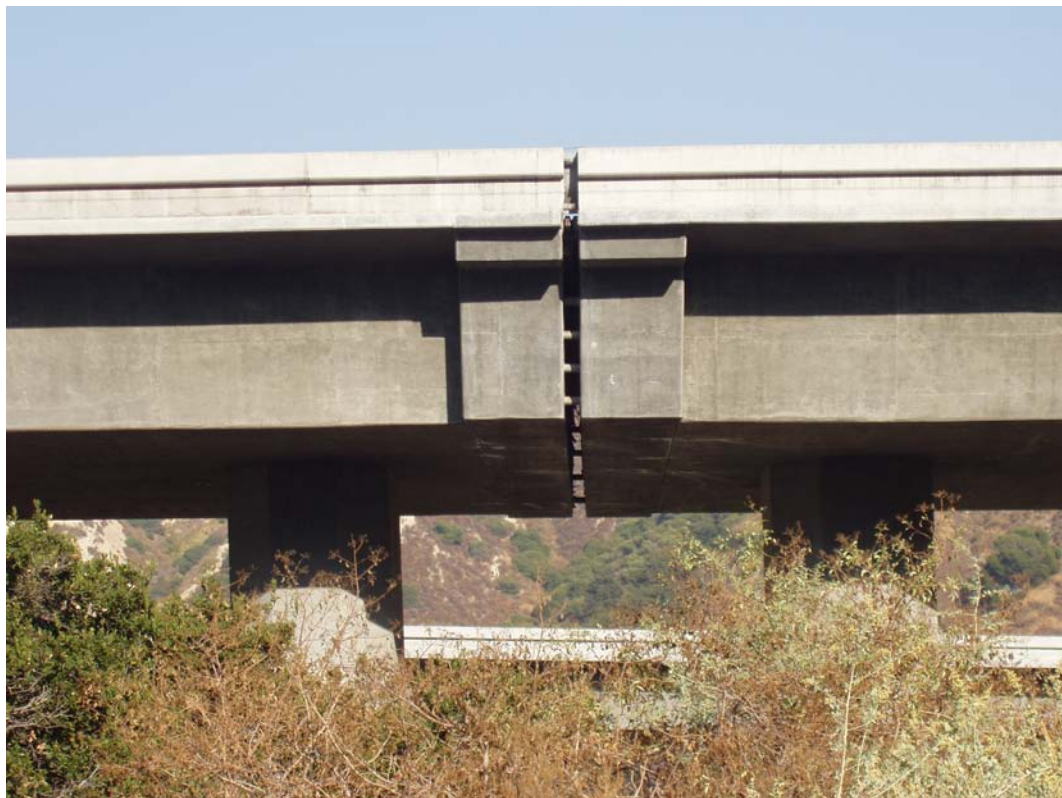
Figure 4. North Connector, looking east at hinge detail.
