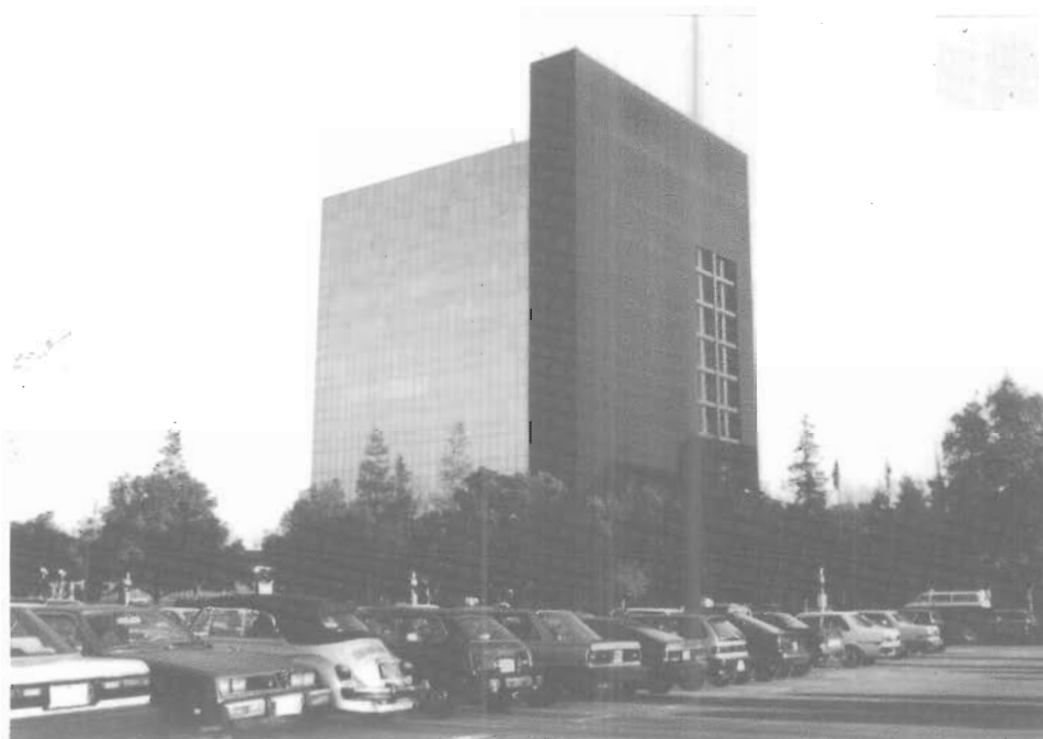
Figure 2: Santa Clara County Government Center - San Jose Overall View from the North-West
