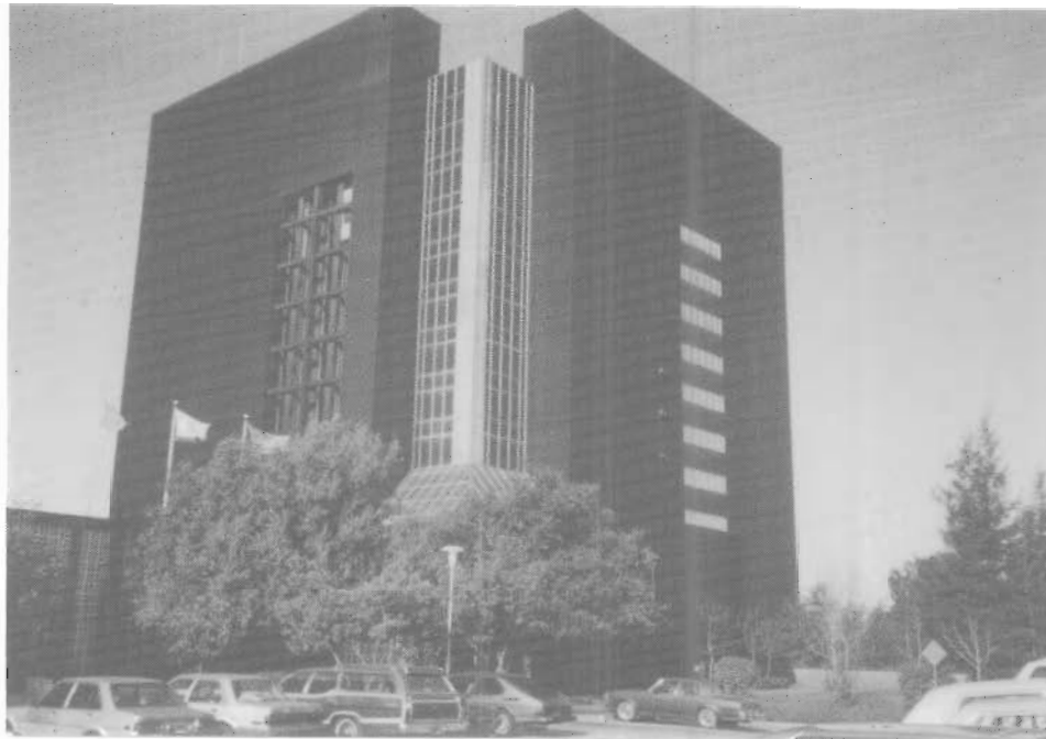
Figure 1: Santa Clara County Government Center - San Jose Overall View from the South-West
