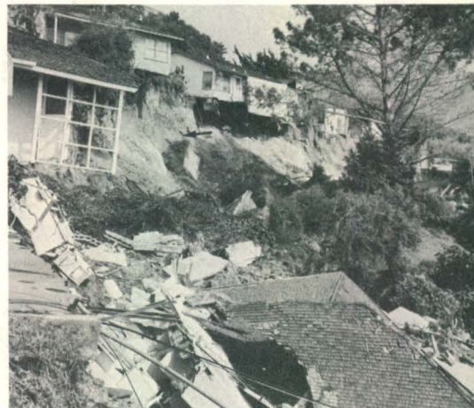
Photo 1. Closeup of headscarp, looking northeast. Arrow pointing to area above concrete slab shows where evidence of older slide plane was found. Exposed bedrock in the headscarp is silty sandstone of the Miocene Topanga Formation. Photo courtesy City of Laguna Beach.
