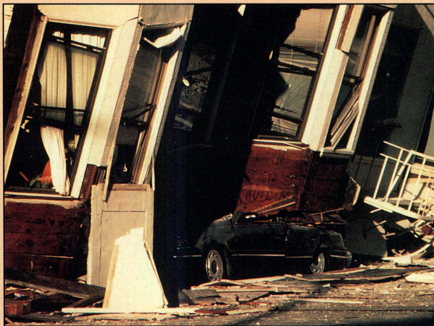
An automobile lies crushed under the third story of this apartment building in San Francisco's Marina District. The first two stories are no longer visible because of structural failure and sinking due to liquefaction, the transformation of the soil from a solid to a liquid state. Photo by John Nakata, U.S. Geological Survey.
