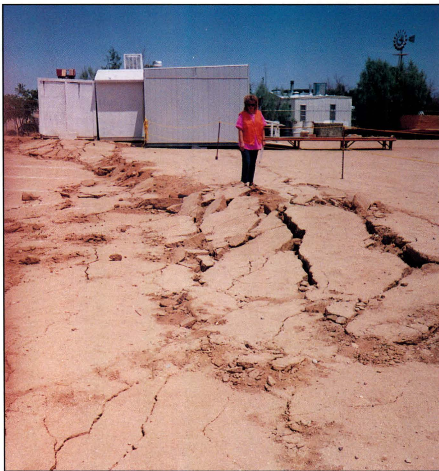
Main trace of Johnson Valley fault at the Country Gospel Church in the Flamingo Heights area. Zone of fracturing is approximately 30 feet (10 m) wide. More than 6 feet (2 m) of right lateral displacement was measured at the parking spaces (upper left). Photo by Jack McMillan.
