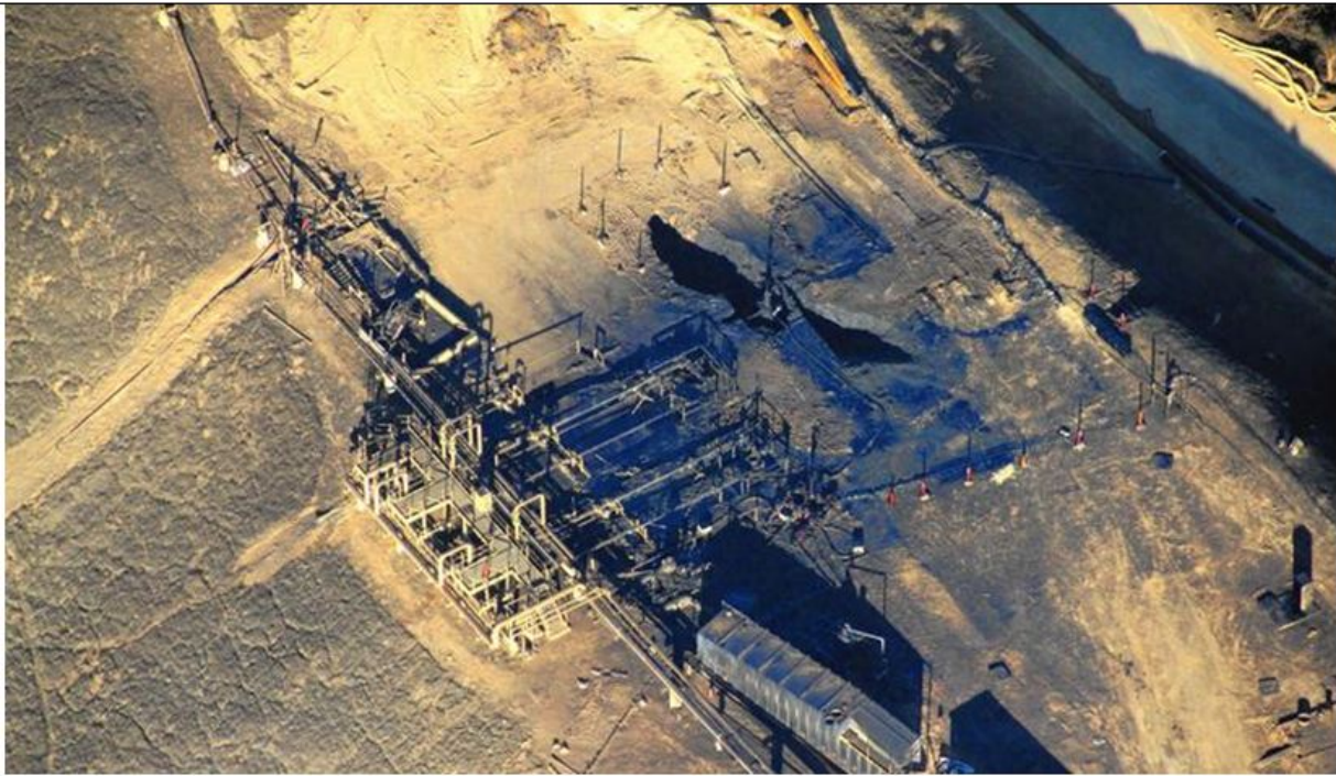
Figure SB-2. The SS-25 wellhead is shown in the upper right-hand quadrant of this image along with the two craters extending diagonally from the well in the photo. Source: http://www.latimes.com/local/california/la-me-aliso-well-hole-20160115-story.html (Accessed 7/30/17).
