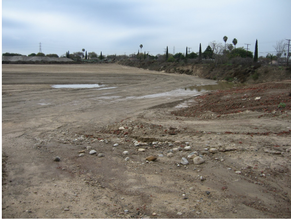
Figure 3. Atkinson Pit No. I located in the City of Compton. This former open pit clay mine is being reclaimed via backfilling to the adjacent street level for industrial land use. (Photo credit: Will Arcand)
