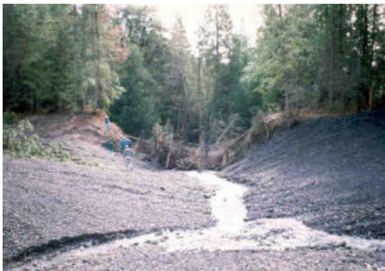
When this log tailings dam at the Lava Cap Mine failed in 1997, it released arsenic laden tailings into Clipper Creek.
