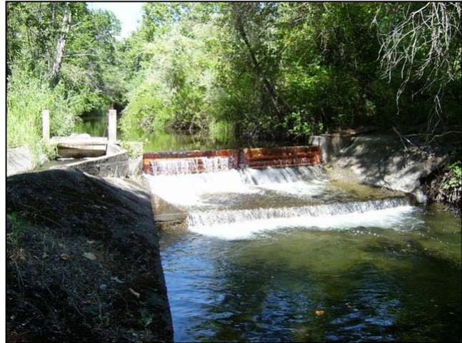
*The Cone-Kimball Diversion Dam will soon be reconstructed with a fish ladder. This will allow fish to reach the water above the dam during periods when irrigation diversions occur.*
