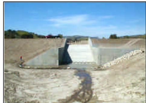
*Grade Control Structure that was designed and built by the RCD on the Santa Rosan Creek*
