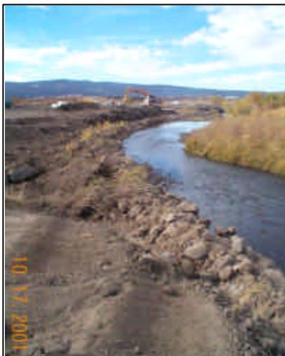
*"Flournoy Project": Longitudinal Stone Toe Production provides protection for new meadow and substrate*
