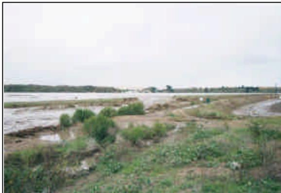
*Arroyo Grande Creek control channel breached, partly due to blockage from accumulated sediment.*
