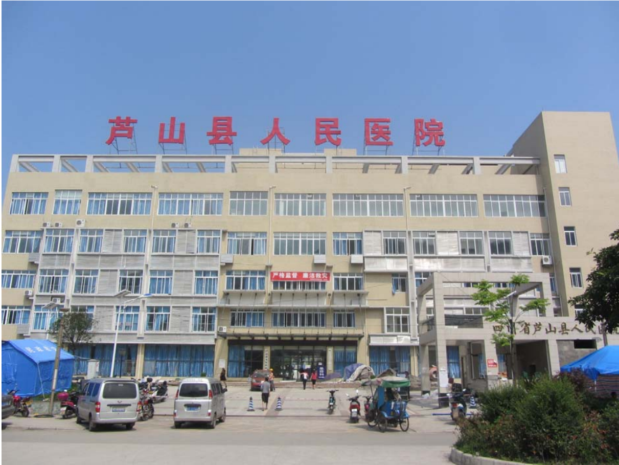
Fig. 17. Base-Isolated Lushan County People's Hospital Outpatient Building. Photograph courtesy of Dr. Craig A. Davis.
