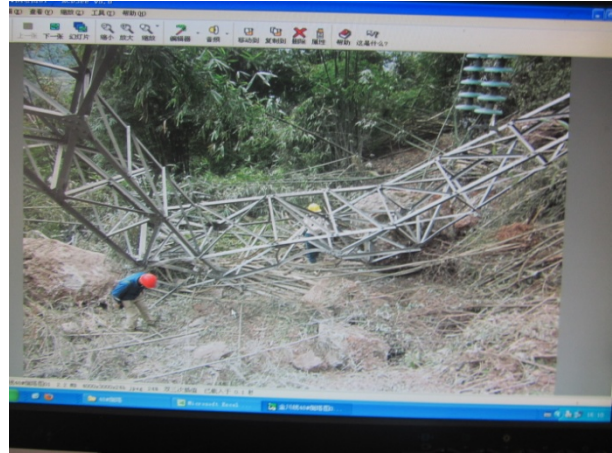
Fig. 24. Transmission tower collapse. (Photograph by Dr. Craig A. Davis)
