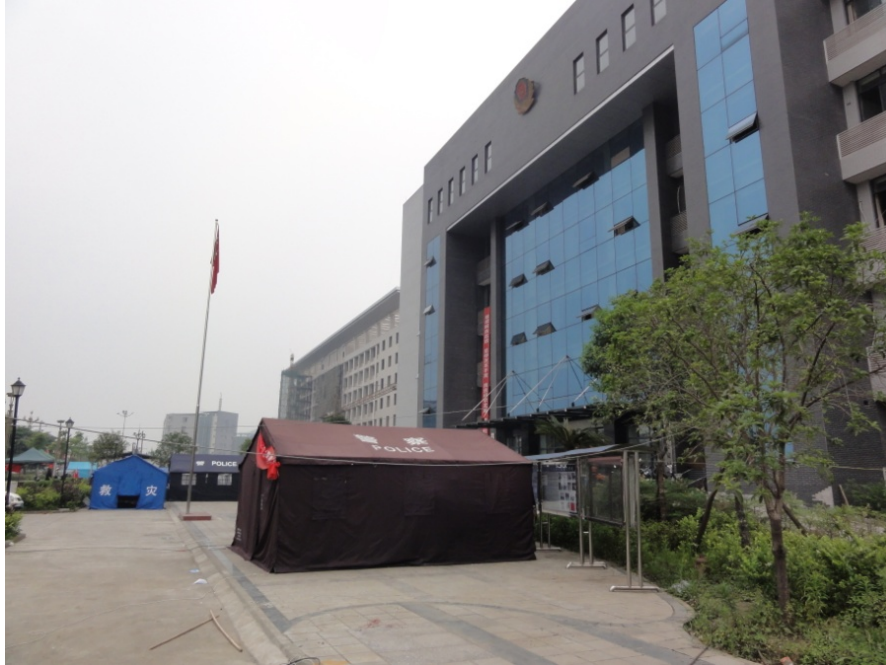
Fig. 13. Relatively new government building in New Lushan Town.
