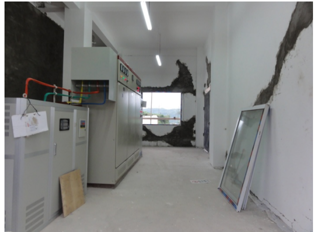
(b) Interior of control building
