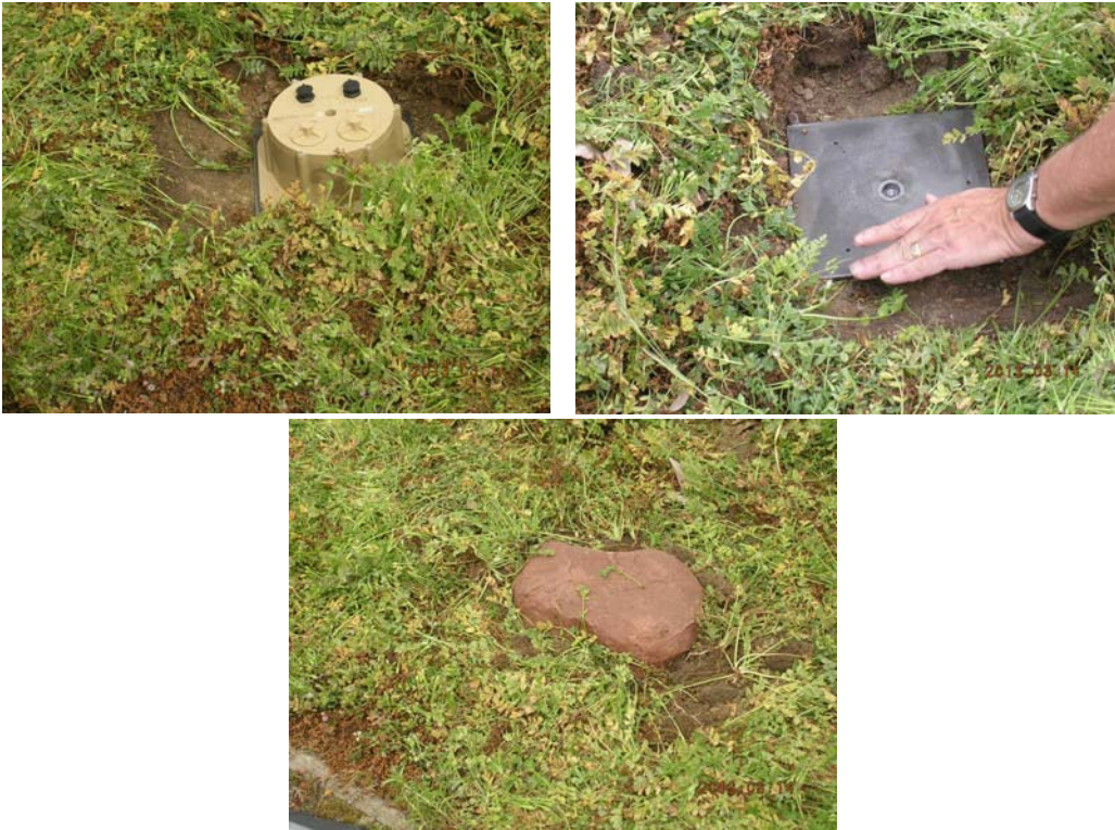
Fig. 8. Illustration of the installation of a QuakeRock accelerograph in a roadside environment. The instrument is shown at upper left (RefTek's 148-01 accelerograph), attached to the mounting plate (upper right), which is attached to an anchoring rod driven into the ground. The finished deployment at bottom shows the faux rock cover over the instrument. The instrument operates autonomously on the included D-cell lithium batteries for up to two years.
