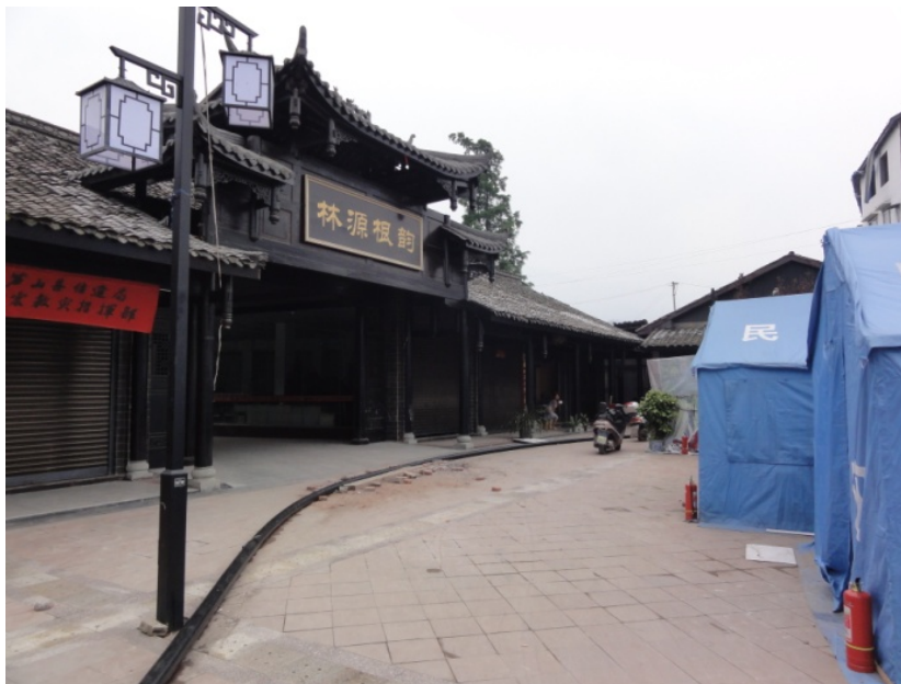
Fig. 19. Temporary above ground water pipe (foreground).
