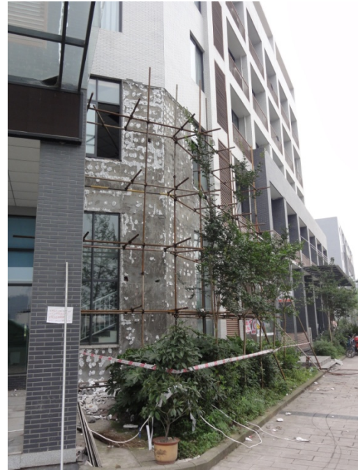
(b) Damaged exterior tiles removed
