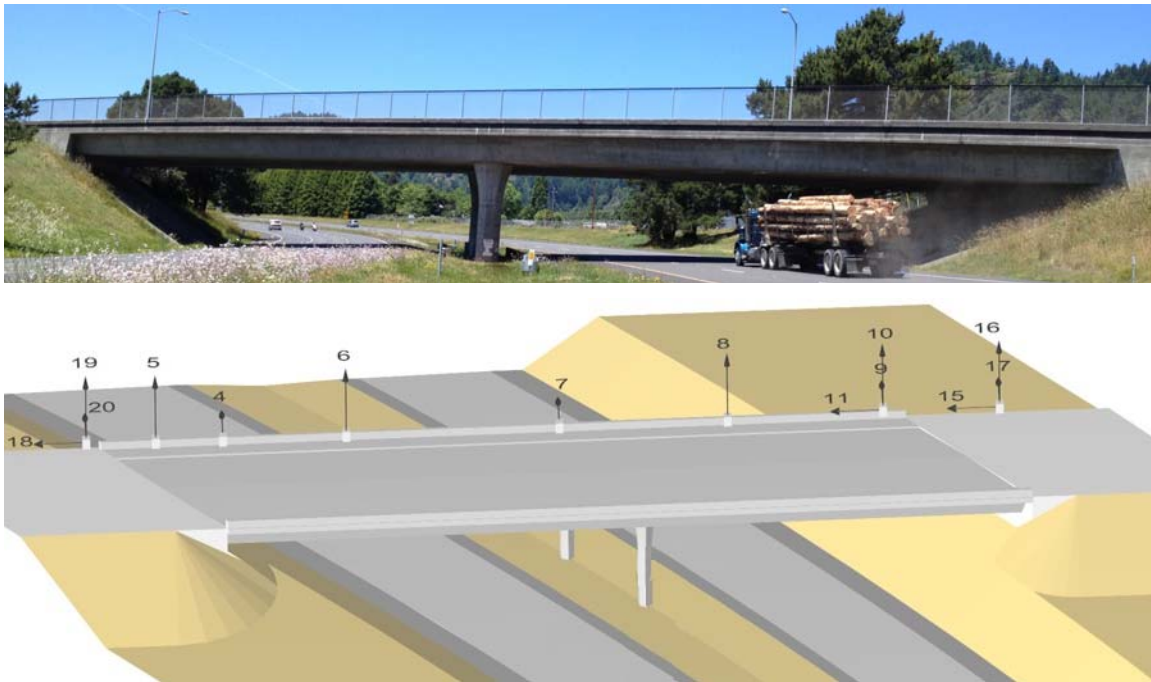
Figure 3. The Painter Street Overpass (top) and its seismic instrumentation (bottom).
