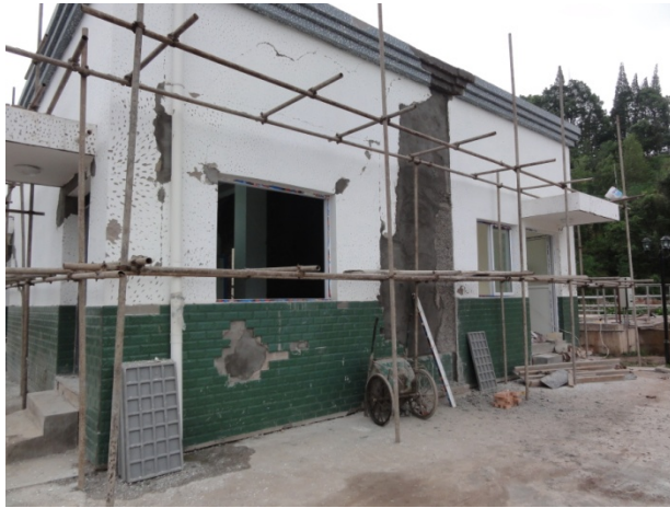
(a) Exterior of control building
