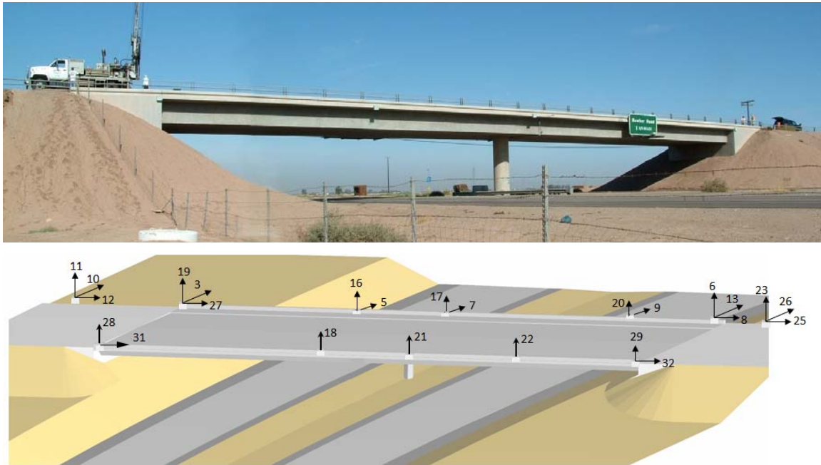
Figure 1. Meloland Road Overcrossing (top) and its seismic instrumentation (bottom).
