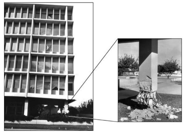
Figure 2. Photos of south face (left) and failed reinforced concrete column (right) at base of Imperial County Services Building, which was damaged by the 1979 Imperial Valley Earthquake. The burst of high frequency motion occurring simultaneously with column failure is shown in Figure 3 (from Rojahn and Mork, 1982).
