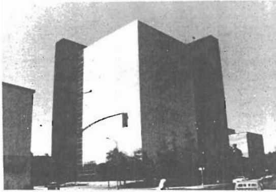
(a) Santa Clara County Office Bldg. 13-story steel frame
