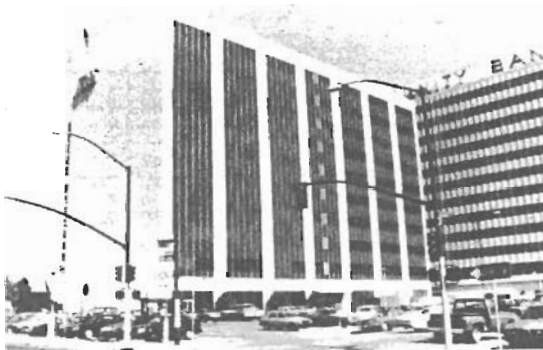
(c) Great Western Savings & Loan Bldg. 10-story reinforced concrete frame and shear walls
