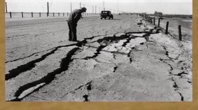
Liquefaction lateral spread lamaged road near Seal Beach.
