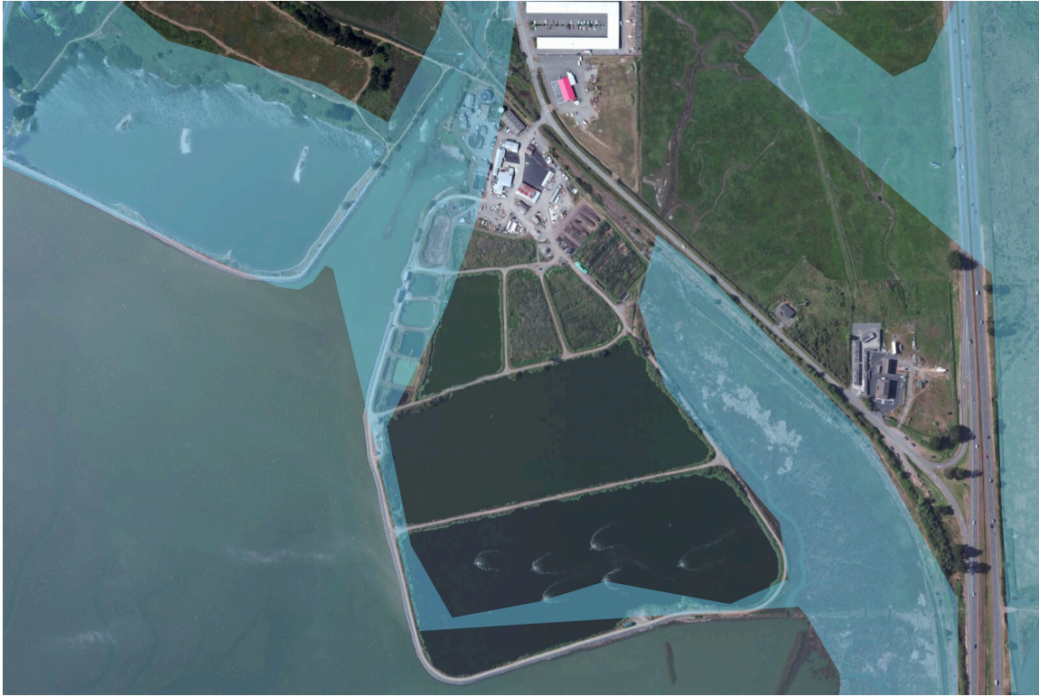
Figure 9. This satellite image shows a wastewater treatment plant indicated to lie partially within the scenario tsunami inundation zone (transparent blue-green). The entire area of the image lies within the California Emergency Management Agency (Cal OES) maximum inundation zone.
