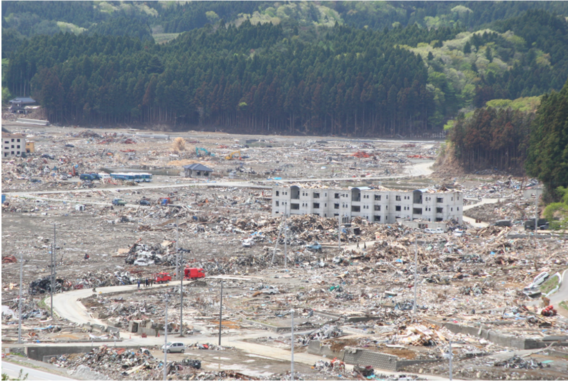
Figure 1. Photograph of the damages caused by the massive tsunami generated by the March 2011 Tohoku earthquake that devastated the northeastern coast of Japan, taken in May 2011 in the Sanriku area. Few buildings were left standing, and extensive debris deposits were left behind. Also note the dying trees at the base of the hills in the background, which were closest to the tsunami inundation area—these were presumably suffering the effects of salt water poisoning. The California scenario tsunami would not cause nearly as extensive or complete devastation as seen in Japan, but would likely cause some damage to buildings in the inundated areas, and leave behind debris. Photograph by Bruce Jaffe, U.S. Geological Survey.
