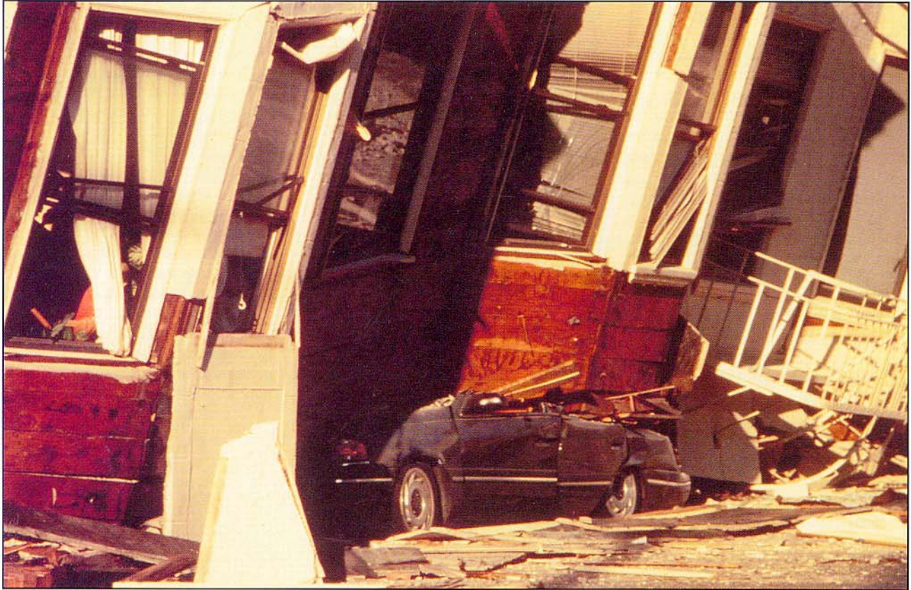
An automobile lies crushed under the third story of this apartment building in San Francisco's Marina District. The first two stories are no longer visible because of structural failure and sinking due to liquefaction, the transformation of the soil from a solid to a liquid state. Loma Prieta earthquake, October 1989. Photo by John Nakata, U.S. Geological Survey.
