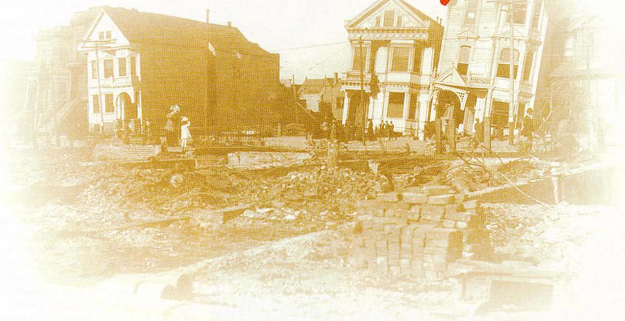
Damage caused by the 1906 earthquake in San Francisco. California Department of Conservation, Division of Mines and Geology file photo.
