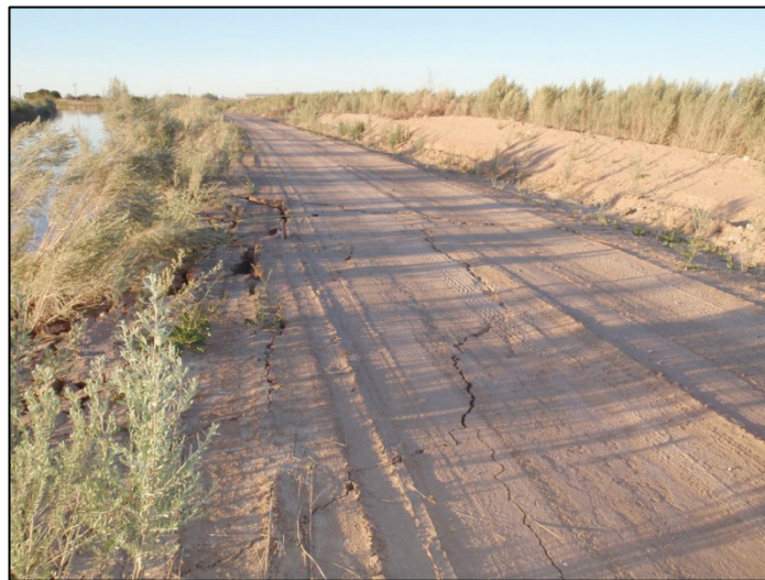
Figure 42. View to north across inferred liquefaction lateral spread in the east bank of the Westside Main Canal (C14). Extensional fractures are open to 95 cm depth and extend across entire width of Westside Main Canal east service road for tens of m. Photo by J. Tinsley, 4/6/10.
