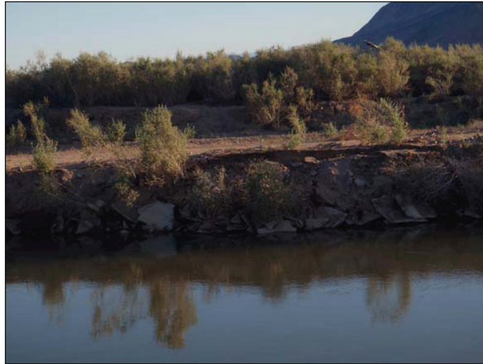
Figure 41. Bank failure probably unrelated to liquefaction in the west bank of Westside Main Canal (C08). This style of failure was observed on both sides of the Westside Main Canal for nearly a kilometer north of State Highway 98. Failures seldom extended more than a meter or two into the levee materials and the bulk of the levees remained undamaged. Photo by J. Tinsley, 4/7/10.
