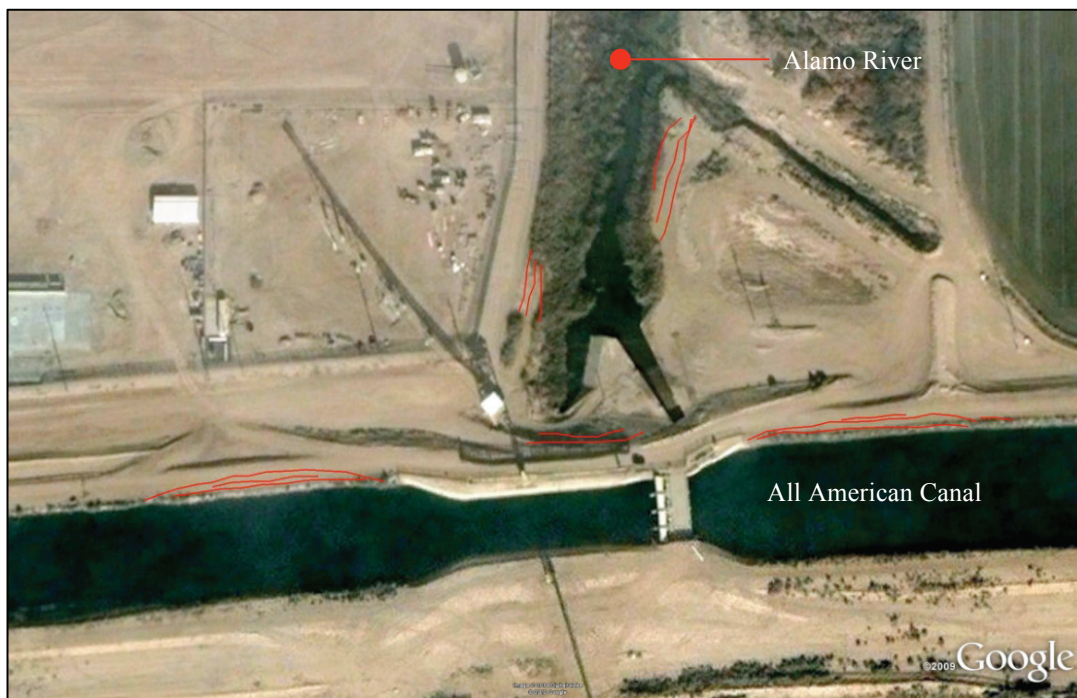
Figure 64. Diagrammatic sketch of cracks and fissures observed on the north side of the All American Canal where it crosses the Alamo River (C55). The Alamo River flows to the north beneath the canal. Base Image is from Google Maps.
