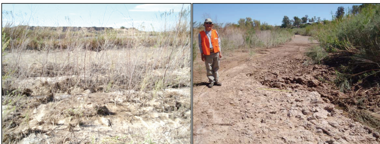
Figure 82. Depositional and erosional features resulting from seiche wave overtopping of Fig Lagoon levee (D10). A, Sand deposition and flow features on the Fig Lagoon levee as a result of overtopping by seiche waves. Water flow came toward the photographer. Lateral spread slump is in the middle background; Fig Lagoon is beyond riparian vegetation on the outer edge of the slump. Photo by T. McCrink, 4/10/10. B, Outwash channel eroded into the Fig Lagoon levee adjacent to the New River. Lateral spread slump shown in figure 80 is immediately left of this photo, and the New River is immediately to the right. Photo by J. Tinsley, 4/7/10.
