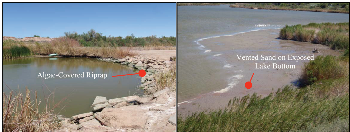
Figure 84. Zone of liquefaction-triggered ground failure in Fig Lagoon levee 175 m north of the slump and overflow channel depicted in preceding photos (D10). A, Scarps in the levee indicate that differential subsidence into a liquefied substrate probably occurred. B, Sand boil deposits presently underwater atop late Holocene floodplain deposits of New River at Fig Lagoon. Preservation of vented materials is morphologically excellent, indicating that a subaqueous eruption is probable. Photos by J. Tinsley, 4/7/10.
