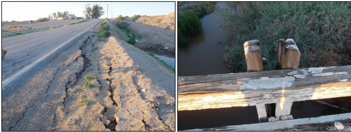
Figure 5. A, View along east margin of Brockman Road near Greeson Drain (R02) showing fractures and slumping of road fill. Tape in middle ground is 1 m long. Extensional cracking also affected pavement of Brockman Road. B, Strong ground shaking and ground deformation in fill drove the wood guardrail from south to north, causing posts supporting the guardrail to split. Photos by J. Tinsley, 4/7/10.
