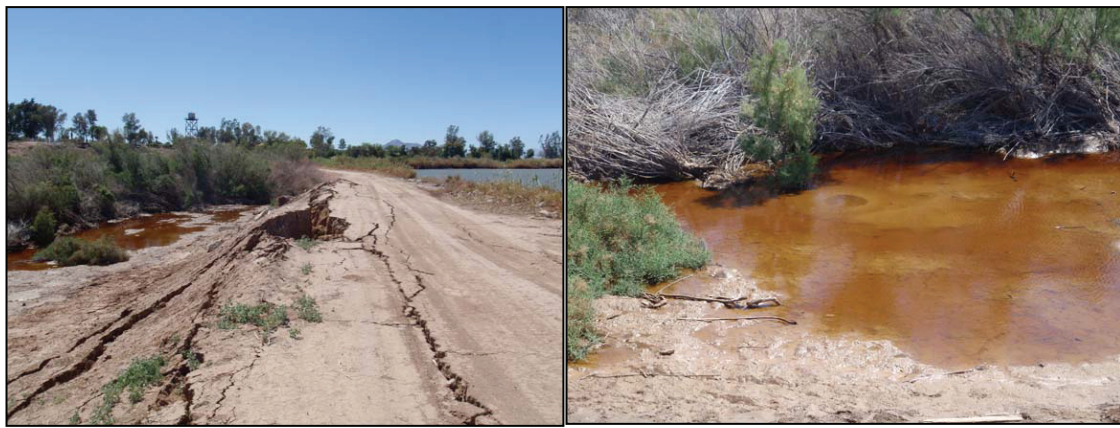
Figure 84. Zone of liquefaction-triggered ground failure in Fig Lagoon levee 175 m north of the slump and overflow channel depicted in preceding photos (D10). A, Scarps in the levee indicate that differential subsidence into a liquefied substrate probably occurred. B, Sand boil deposits presently underwater atop late Holocene floodplain deposits of New River at Fig Lagoon. Preservation of vented materials is morphologically excellent, indicating that a subaqueous eruption is probable. Photos by J. Tinsley, 4/7/10.
