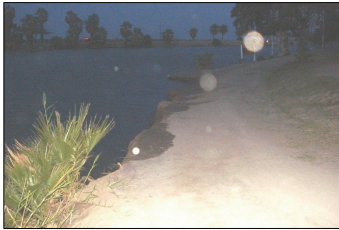
Figure 105. Photograph of the south bank of Sunbeam Lake (F02). Wet areas, shown as dark soil at the edge of the dirt path, indicates where water splashed out of the lake. The steep sides of the bank are on the order of 0.5 m high. Photo courtesy of Imperial County Parks and Recreation; taken 4/4/10.
