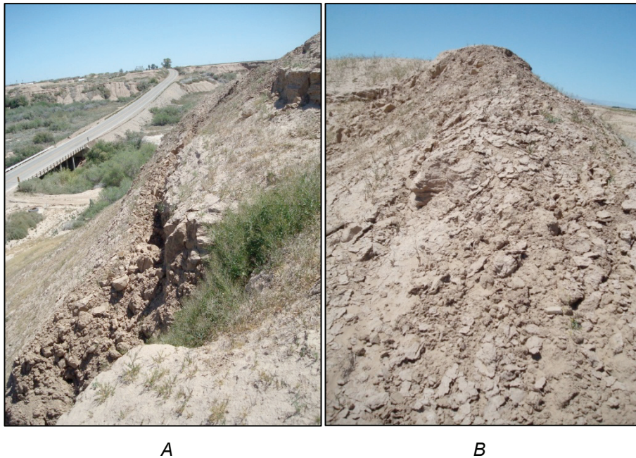
Figure 27. Slope effects near the top of the New River bluff at the Keystone Road Bridge (R23). A , View of Keystone Road Bridge at the New River with detached mass of colluvial soil in foreground. View to the northeast. B , Shattered soil crust on small east-west ridge southwest of the Keystone Road Bridge. Photos by T. McCrink, 4/8/10.
