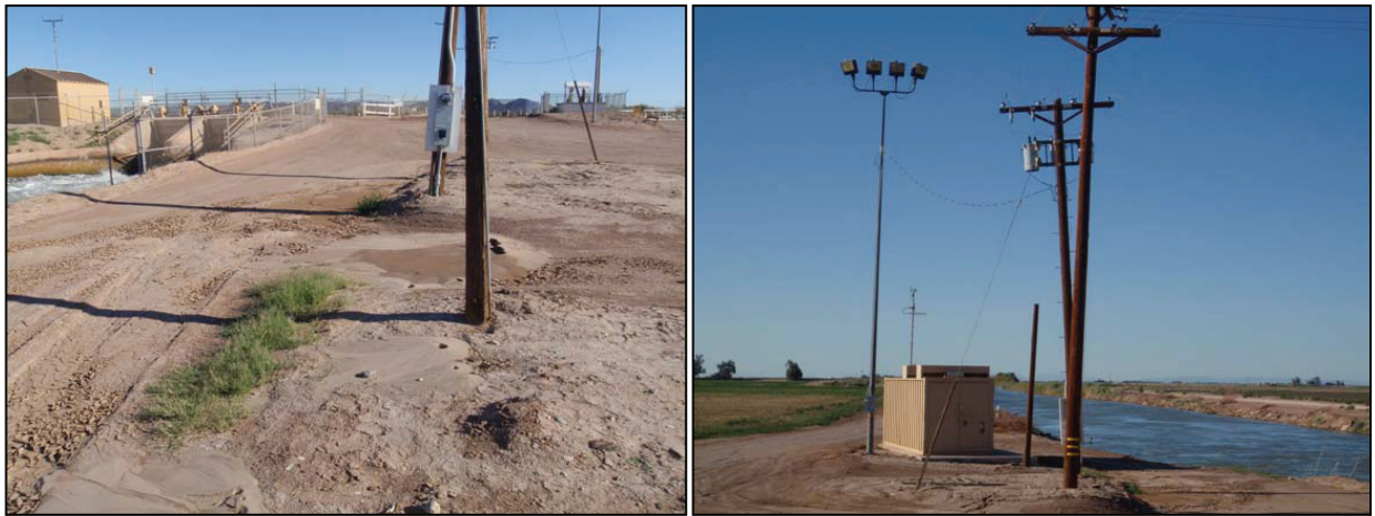
Figure 32. View north along west bank of Westside Main Canal, showing utility poles tilted from plumb due to lateral spreading ground failure (C01). Area around base of poles shows light-toned vented sand. Venting of sand in proximity to the poles probably reflects soil-structure interaction that enhanced liquefaction. Photos by J. Tinsley, 4/6/10.
