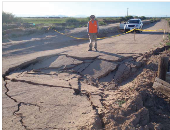
Figure 38. Collapse of the Westside Main Canal's western access road (C05). Undermining of the road surface probably reflects pre-earthquake piping along transverse subgrade structures or other zone of seepage from the canal. No vented liquefied materials were noted in the area. Photo by J. Tinsley, 4/6/10.
