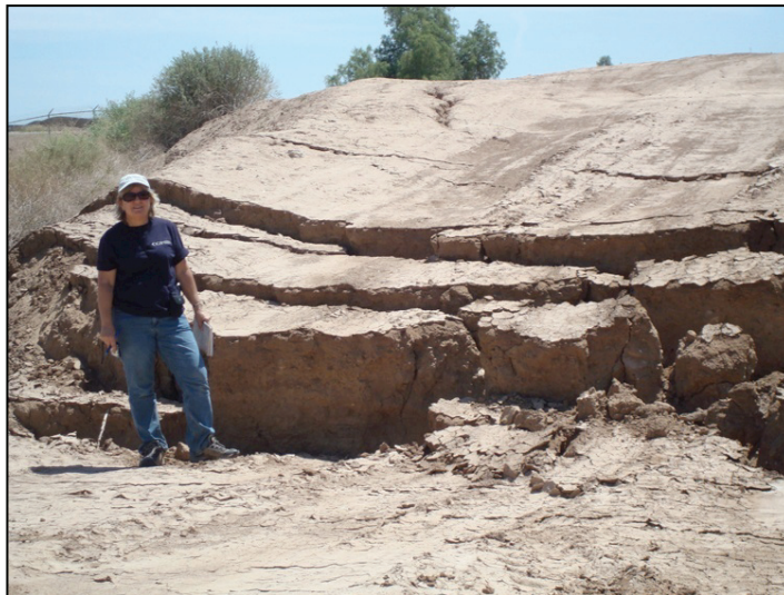
Figure 115. View to the southeast of a large scarp at the head of a liquefaction lateral spread on the west side of the Calxico Waste Water Treatment Plant (F04). Cumulative vertical displacement is about 1 m. Photo by T. McCrink, 4/10/10.
