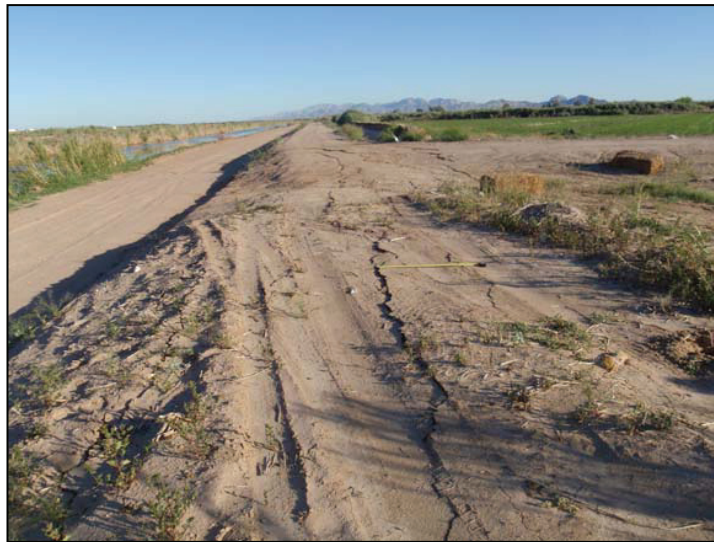
Figure 39. View of extensional fractures at head scarp of lateral spread crossing the embankment in the foreground and including Westside Main Canal's service road to the left (C06). Riparian vegetation is tilted towards the canal owing to lateral spreading. Photo by J. Tinsley, 4/6/10.
