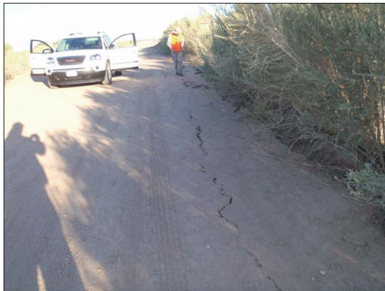
Figure 40. Minor extensional fractures parallel to the channel of the Westside Main Canal (C07). No vented materials were observed in association with this ground failure; the failure is likely a result of strong shaking and not liquefaction. Photo by J. Tinsley, 4/7/10.
