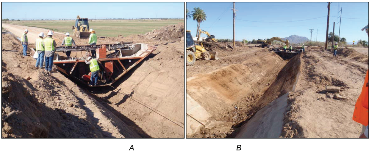
Figure 48. Repairs to the liquefaction-damaged Fern Canal (C29). A , Repair crew adjusts grading equipment to shape walls of the Fern Canal to repair the effects of lateral spread ground failure. B , View to the south with Mount Signal (El Centinela) in the distance, showing reshaped canal prior to pouring new concrete walls and bottom. Photos by J. Tinsley, 4/7/10.
