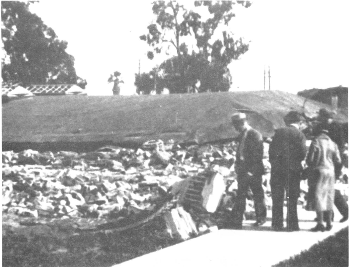
Photograph 4. Collapsed single story business building of unreinforced masonry, in the 1933 earthquake. Photo by Olaf P. Jenkins.
