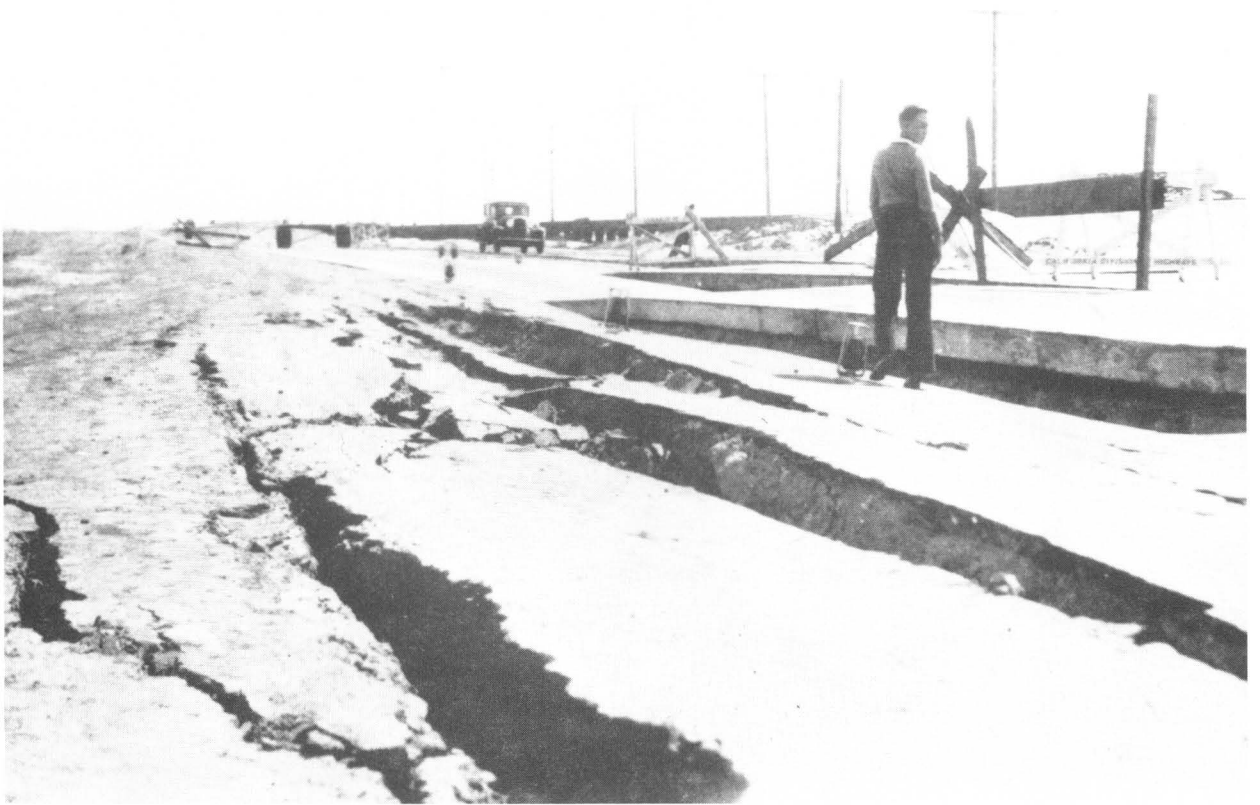
Photograph 8 Settling cracks along Pacific Coast Highway 1.4 miles southeast of Huntington Beach Pier, in the 1933 earthquake. Photo from Long Beach Public Library history collection.
