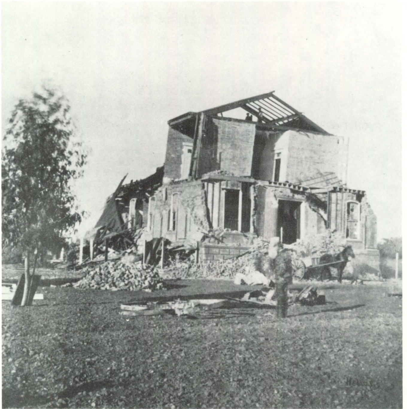
Courthouse at San Leandro after the Hayward earthquake of October 21, 1868.
