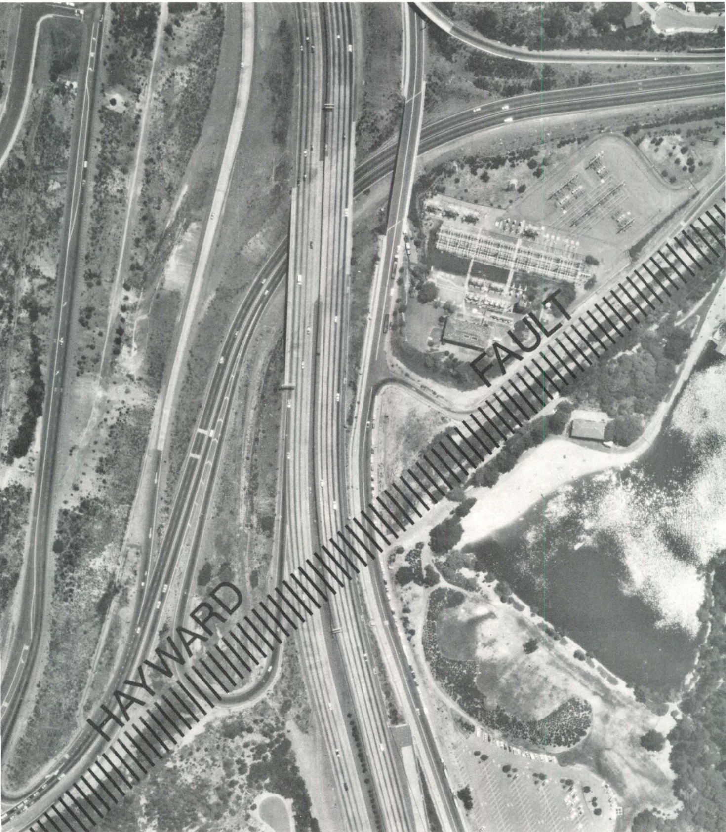
The Hayward fault crossing of Route 24 in the Route 13 interchange area near Lake Temescal and PG & E's Claremont substation.
