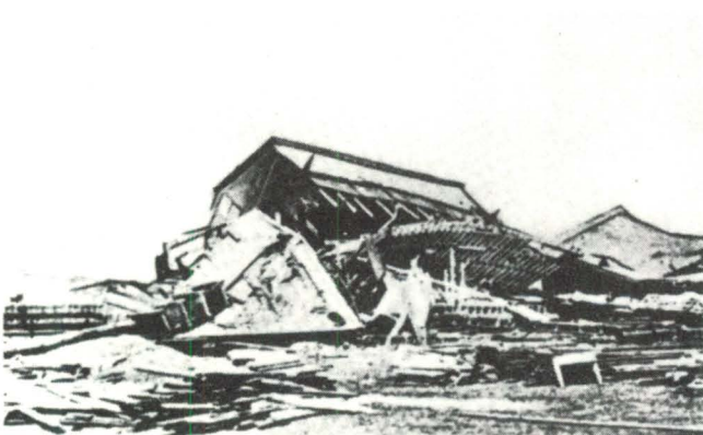
E. Haywards. Wreck of buildings by earthquake of 1868.
