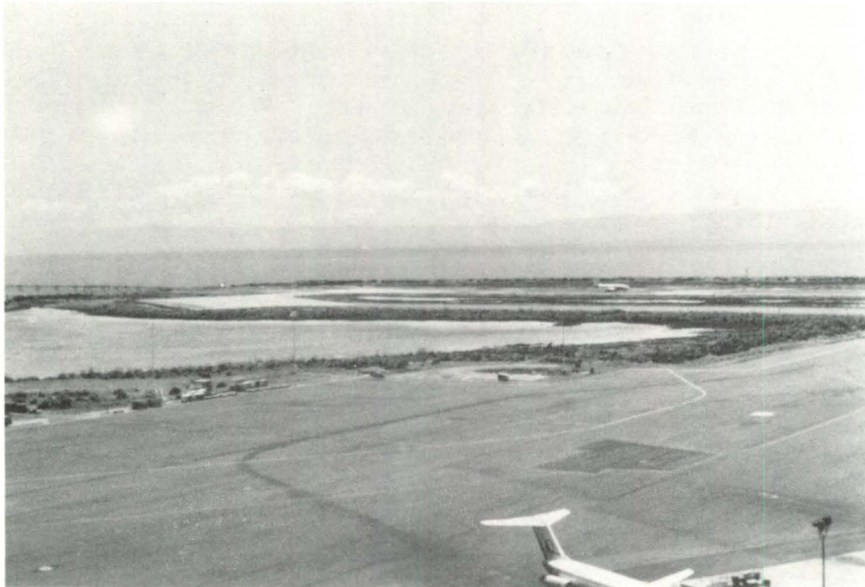
Typical Bay area airport runway constructed on fill overlying potentially unstable soils, including Bay mud.
