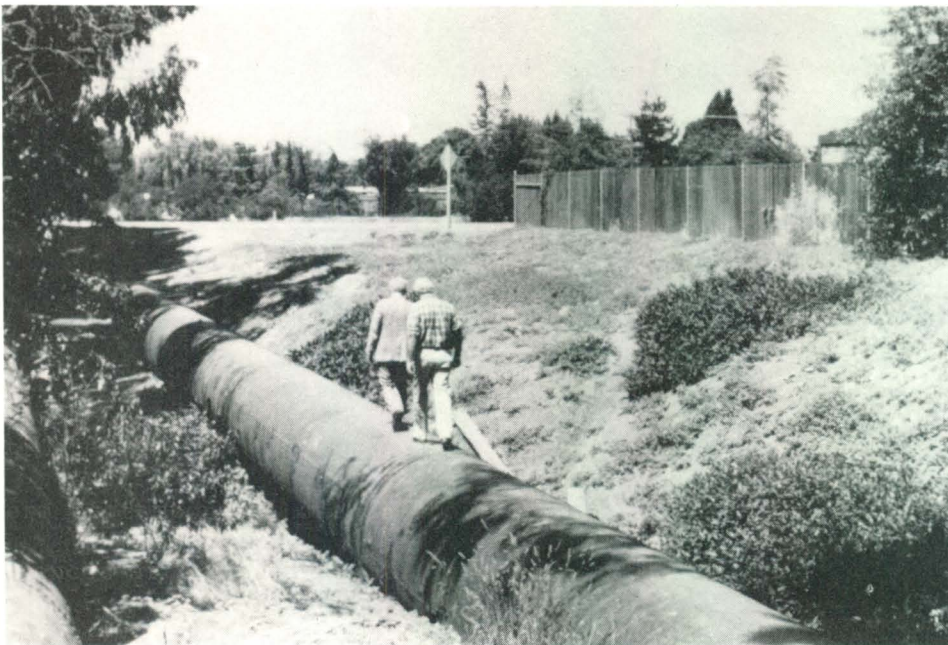
The two trans-Bay Hetch Hetchy pipelines at the Hayward fault crossing in Fremont.
