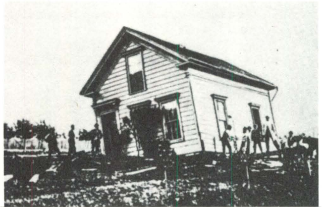
D. Pierce's house, Haywards. Earthquake of 1868.
