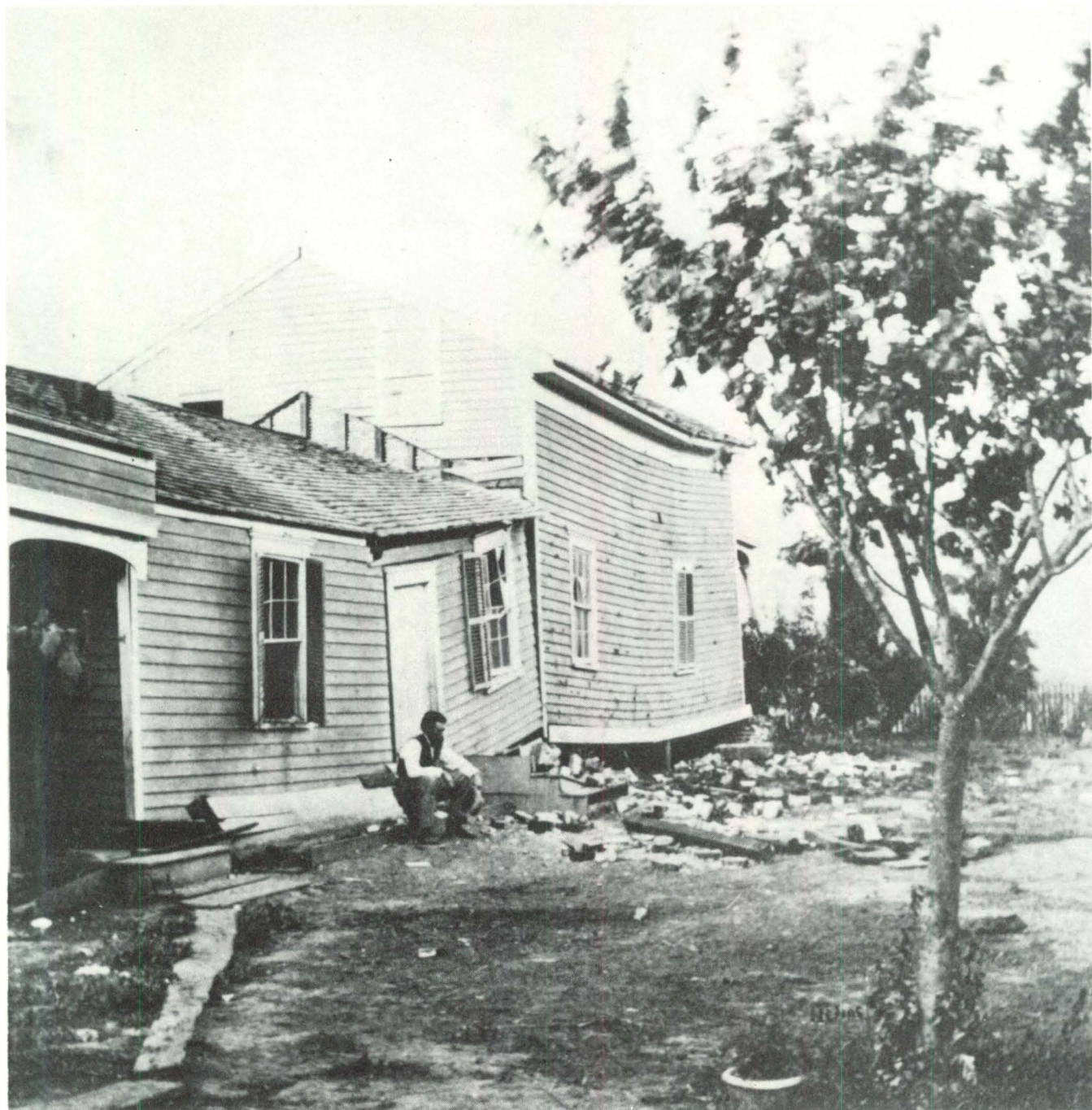
House at Hayward after the earthquake of 21 October 1868. Photo courtesy of the Bancroft Library, University of California, Berkeley.
