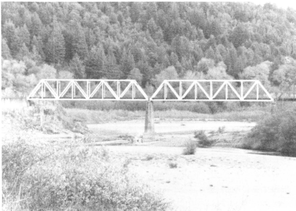
Photo R-1 Railroad bridge across South Fork Eel River at Scotia.
