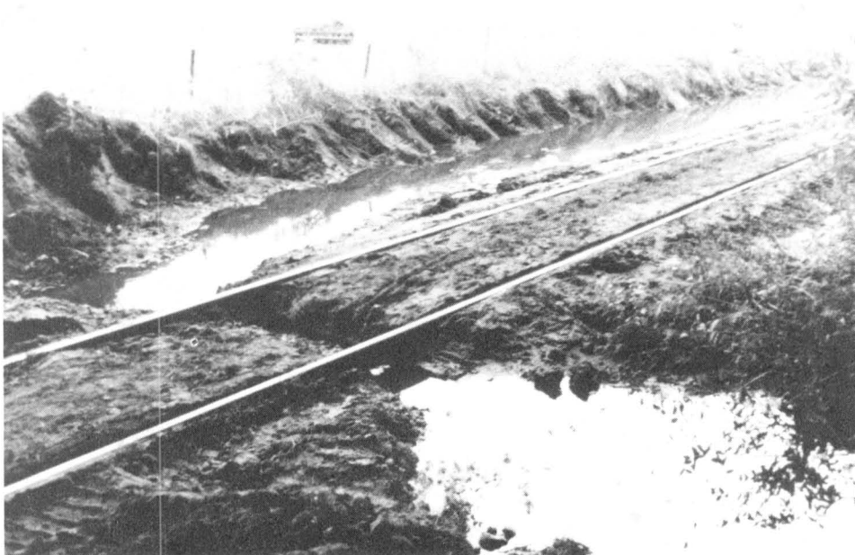
Photo R-2 Railroad tracks beneath Fields Landing overpass.
