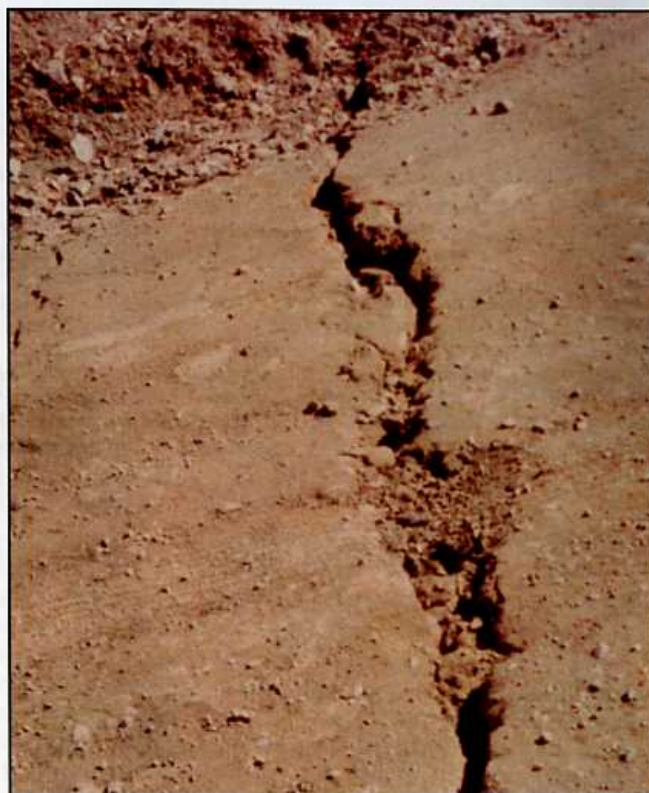
Photo 2. Oriented tensional crack along Wilder Ridge Road, 4 miles (6.4 km) south of Honeydew. Crack orientation is approximately N 30° W, with the downslope side having moved up forming an east-facing scarp. Photos by Robert C. McPherson unless otherwise noted.
