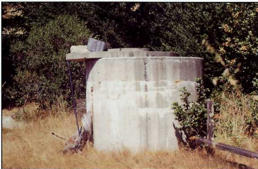
Photo 7. Displaced concrete lid in vicinity of Honeydew. Lid has moved west relative to the tank.
