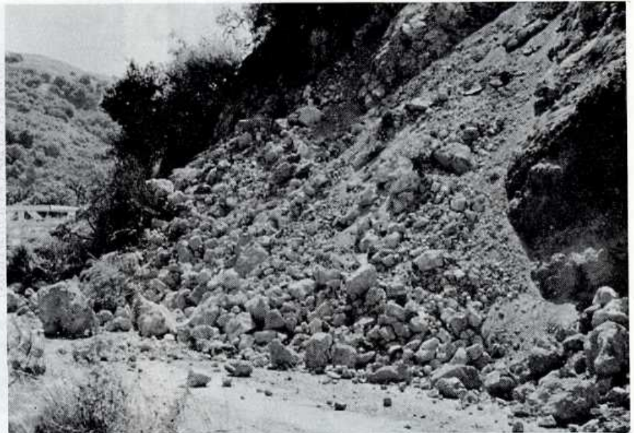
Rockfall at Cockrane Bridge, Morgan Hill earthquake.
