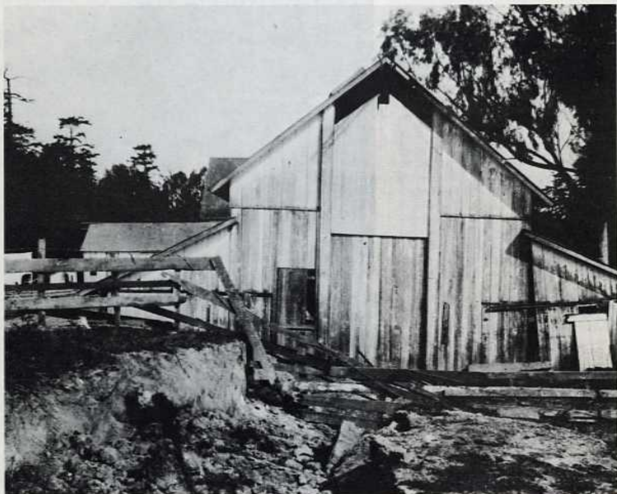
View northwest along the 1906 fault trace towards Skinner Barn. The western portion of the barn remained intact during the earthquake while the southeastern corner was torn 16 feet off its foundation. This barn was reconstructed on the same site in 1940. The barn will be used as a movie theater during the special educational programs that will accompany the earthquake trail dedication ceremonies.
