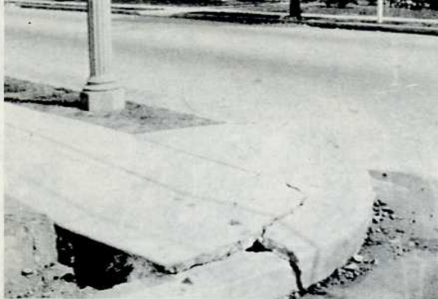
Concrete curb adjacent to the campus of Compton Junior College. Cracks in the curb resulted from motion during the Long Beach earthquake of 1933. Photo by O.P. Jenkins.
