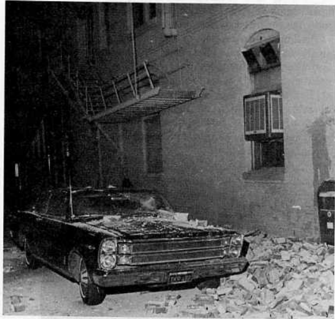
Bricks tumbled from many buildings as a result of the quake. These views of rubble derived from the top of the three-story Galeazzi Building, show successive damage caused by the repeated tremors. The photo in the upper left, taken on the night of October 1, shows damage as a result of the first shock.
