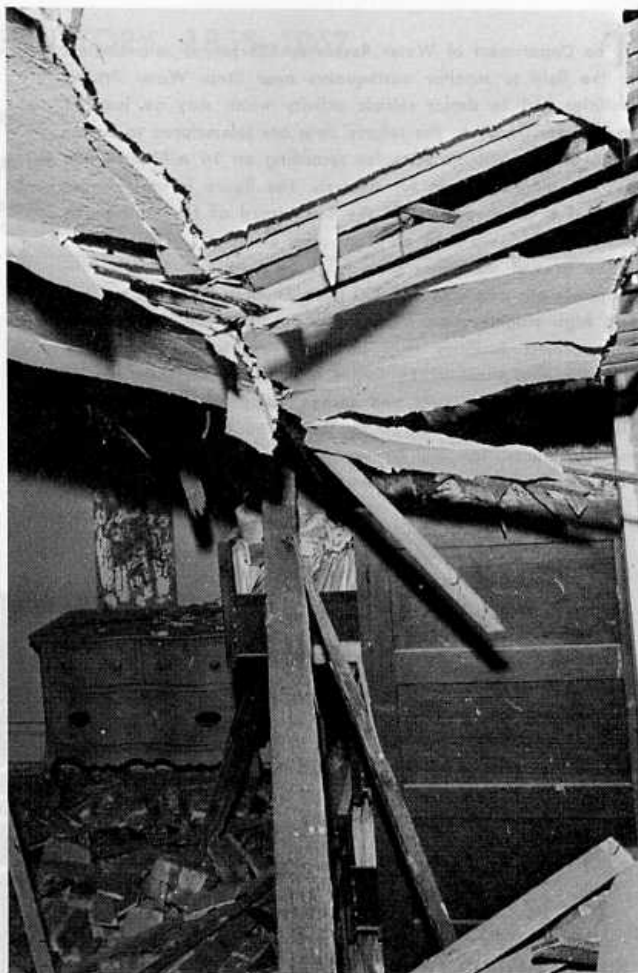
Severe interior damage including collapsed ceiling in office building on College Avenue. Photo by Santa Rosa Press Democrat.
