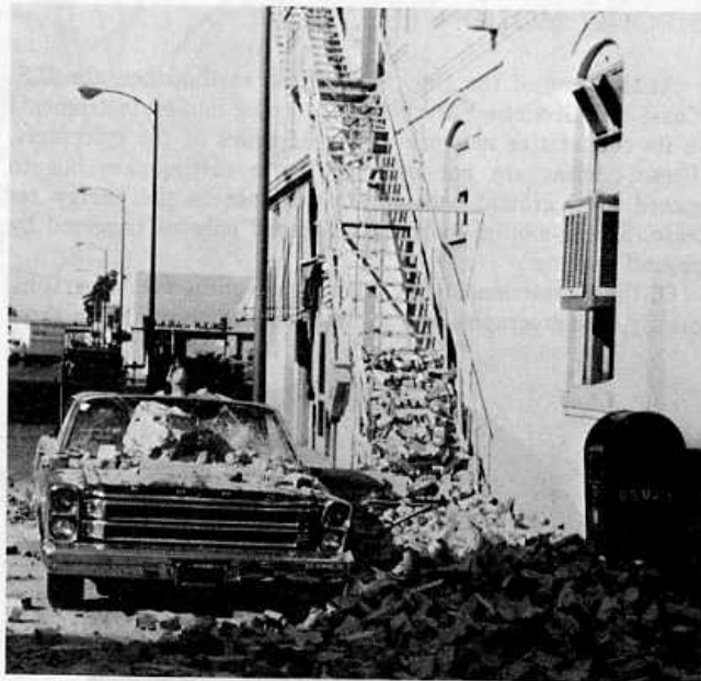
The photo on the upper right, taken the following morning, shows further damage to automobile by falling debris after second strong tremor. The fire escape also dropped, weighted down by added brick. Photo to left by Santa Rosa Press Democrat; to right by Robert D. Nason.
