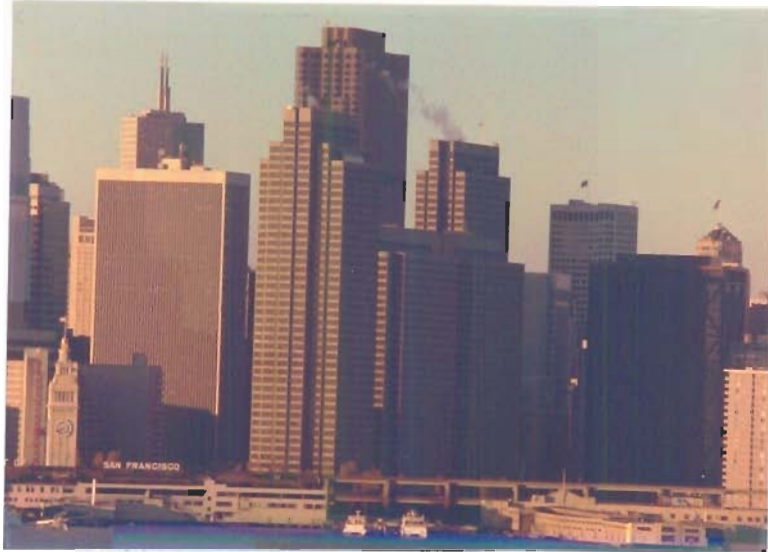
Figure 1. A View of the Structure
