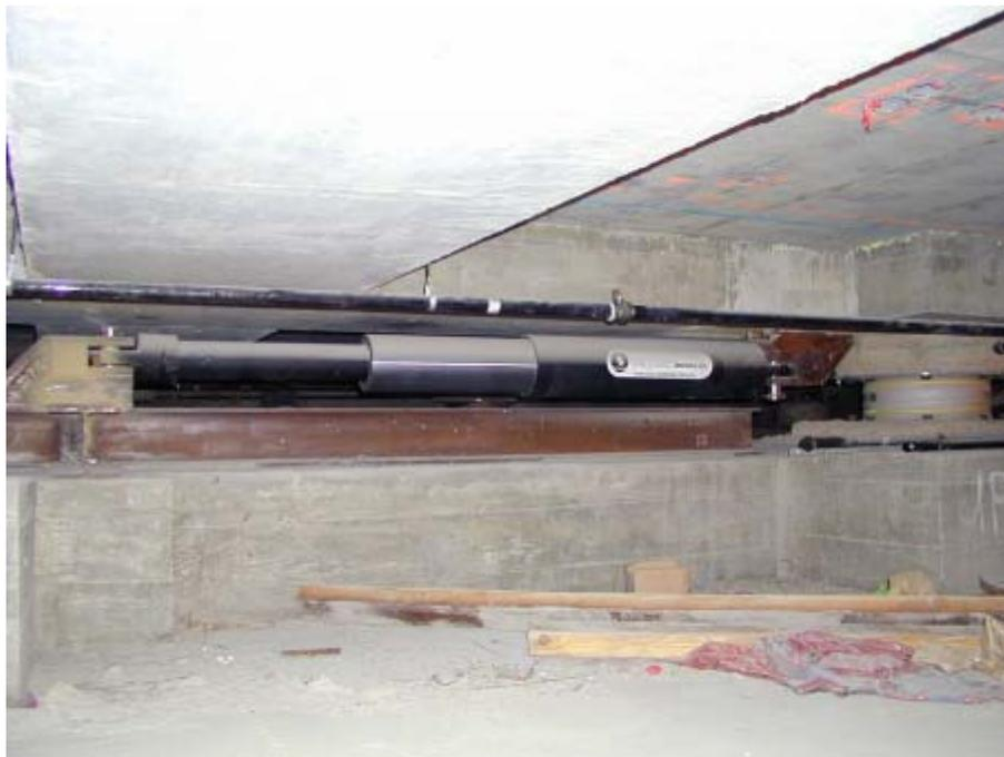
**Figure 10: 300 kip damper installed at plane of isolation**
