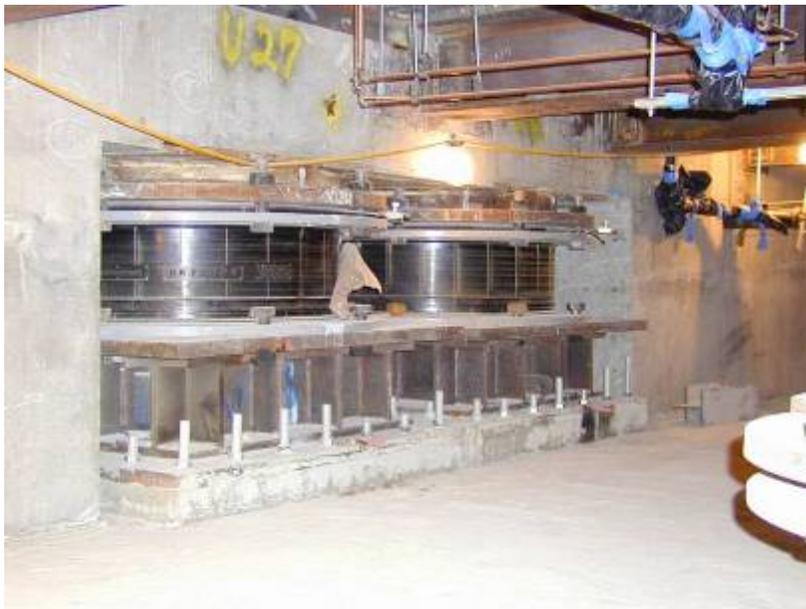
**Figure 8: High damping rubber bearings installed under tower wall**
