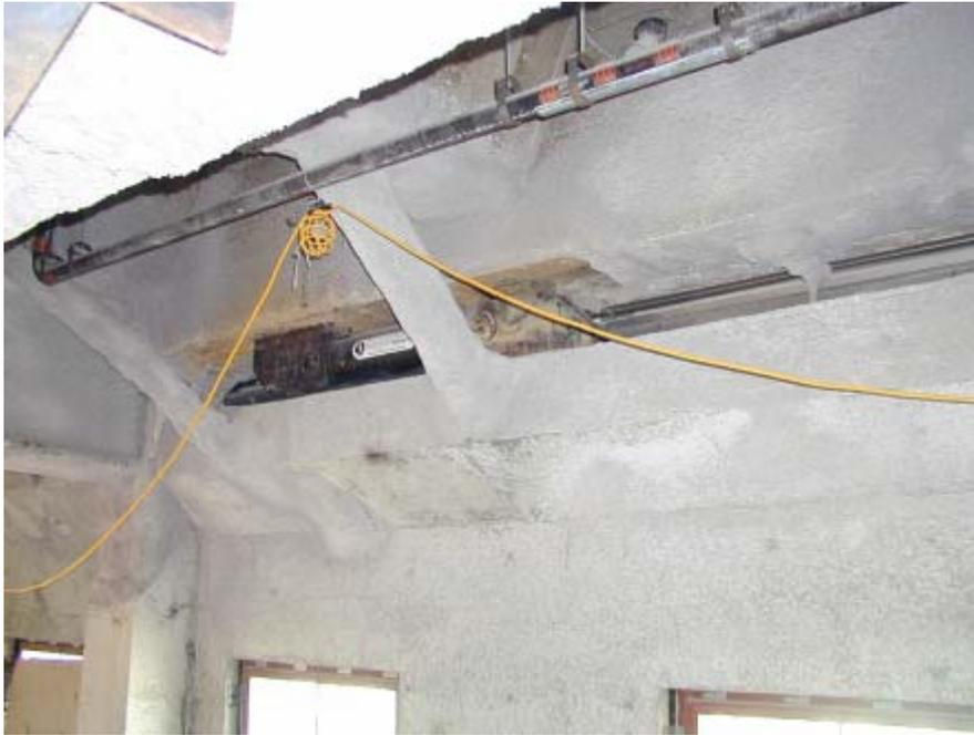
**Figure 11: 225 kip damper installed at 26<sup>th</sup> floor**
