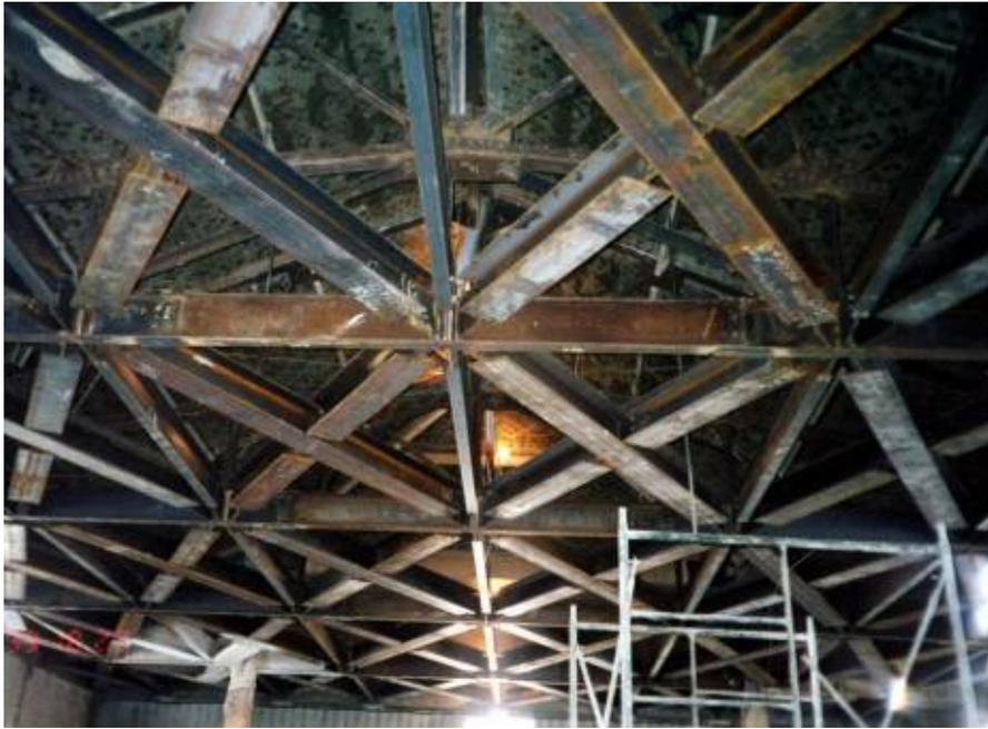
Figure 15: New horizontal steel truss diaphragm at 11<sup>th</sup> floor
