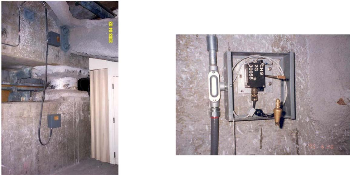
Figure 4. (Left) Sensors 9 (above isolator) and 4 (below isolator) with protecting boxes and conduit installed on the south side of the basement at Oakland City Hall. The cabling has about 2 feet of slack to allow relative movement across the isolator. (Right) Close-up view of Sensor 9 with plumb bob indicating vertical direction.
