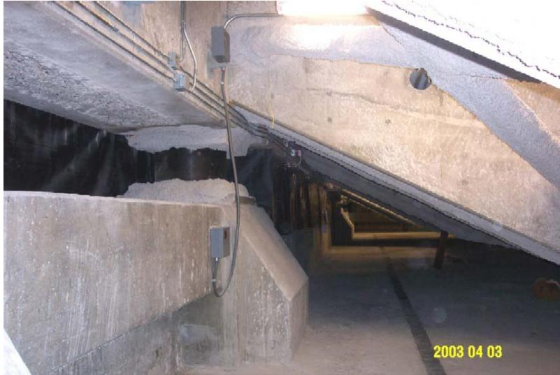
Figure 5. Sensors 7 (above isolator) and 2 (below isolator) with protecting boxes and cabling conduit installed on the east side of the basement at the Oakland City Hall to measure vertical motions.
