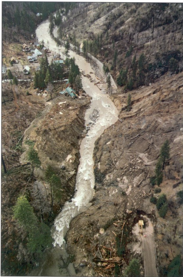
Photo 2. View westward down the South Fork American River showing the breached landslide toe and about 800 lineal feet (245 m) of U.S. Highway 50 buried. Photo by Robert H. Sydnor.
