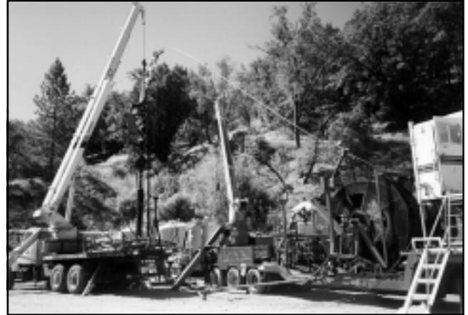
The EPA plugged and abandoned seven hazardous wells on Unit 15 at The Geysers Geothermal field. One was well “Rorabaugh” A-7, pictured here. *Photo by E. Johnson.*
