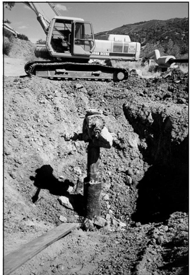
Well “Rorabaugh” A-1, after it was plugged and abandoned on Unit 15. The wellhead was later cut off at the base, near the level of the plank, and buried. *Photo by E. Johnson.*
