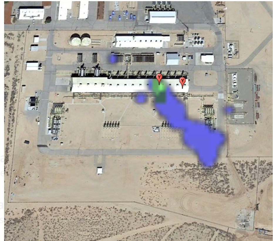
• Leaking natural gas compressor station
