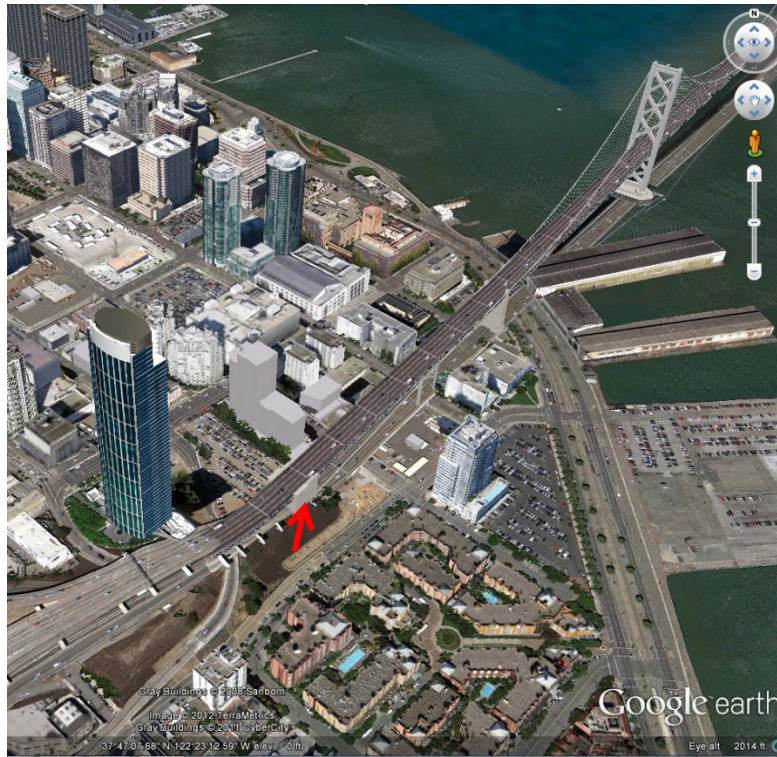
Figure 1. Google Earth ® street view showing the building (left center) and vicinity, and the west end of the San Francisco Bay Bridge (SFBB). Arrow points the west anchorage structure of the SFBB, which is approximately 100 m from the building.
