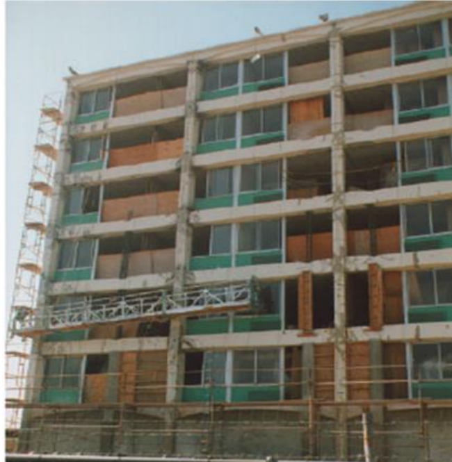
Fig.20: Building site survey during repair works - July 1995, after Lynn et al. [11]
