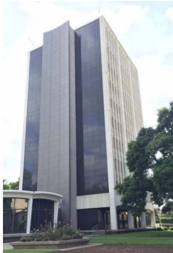
Figure 2: Millikan Library building.
