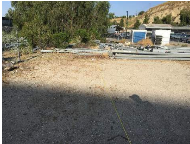
Figure 1 – View of onsite material and limits of survey line tape.
