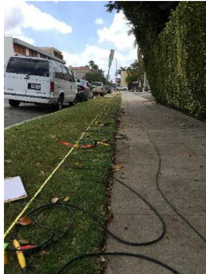
Figure 7 – View of 2D Passive line and general setup.
