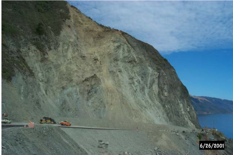
Figure 4, Debris slides above the highway at "Pitkin's Curve" may have formed due to retrogressive failure starting in a road cut.
