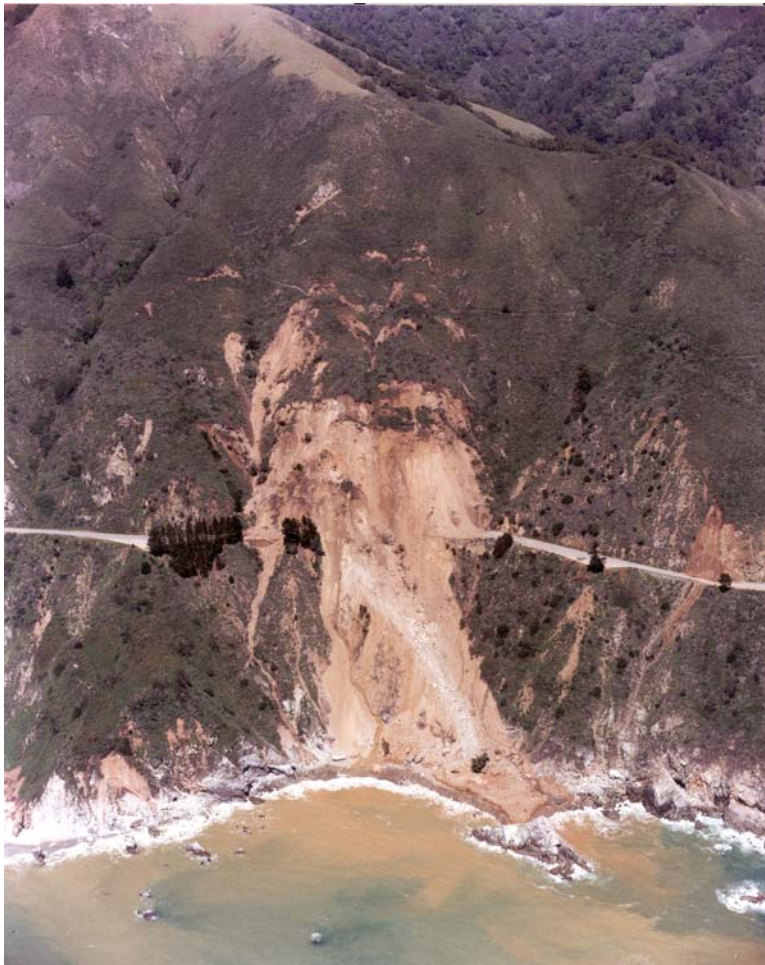
Figure 6. Aerial view of the McWay slide of 1983. Photo by Lynn Harrison, Caltrans
