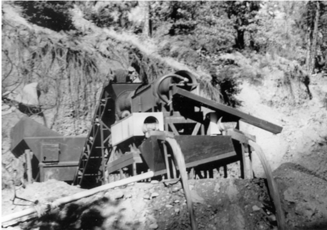
Photo 20. Close up of primary concentrators from Photo 19.
