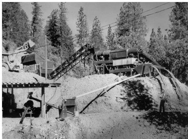
Photo 19. View of TRI-R Engineering's recovery system at the Stinson Mine. Ore is loaded by backhoe into the feed bin, then delivered by conveyor to the trammel. The discharge is coming from the light colored primary concentrators. Concentrates are stored in the sump at left, then processed in the helix.
