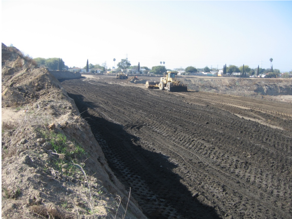
Figure 1. Ongoing fill material placement and compaction in a former Clay Pit that is being backfilled up to original grade in an industrial/residential neighborhood in the City of Compton (Photo by Will Arcand; November 17, 2010).
