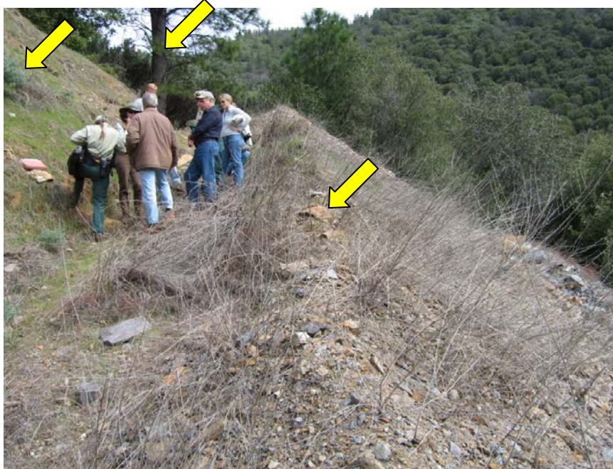
Figure 3. Mine operator, State and County SMARA regulators, and USFS staff standing on haul road traversing the top of a waste rock dump constructed by sidecasting on a steep slope. Arrows point to (from left to right) a lavender bush, pine tree and large rock that are also referenced in Figure 2 (Photo by Will Arcand; March 26, 2006).
