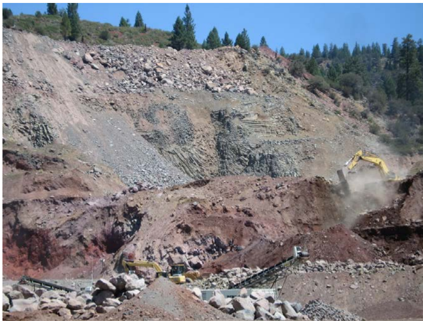
Figure 5. View of quarry cut slope proposed for expansion into volcanic flow rocks of Quaternary age with locally variable structures (columns adjacent to pillows) (Photo by Will Arcand; dated August 2, 2006)
