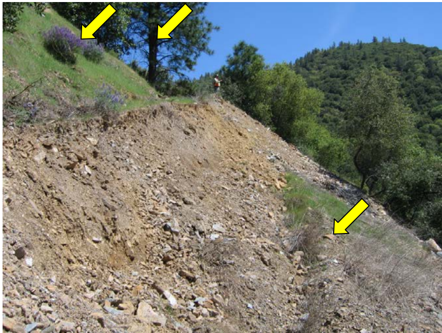
Figure 4. 4/27/06 – Failure of upper portion of waste rock dump approximately one month after photograph used in Fig. 1. USFS staff member visible at upper center. Arrows correspond to reference points described in Figure 1. (Photo by Will Arcand; April 27, 2006)
