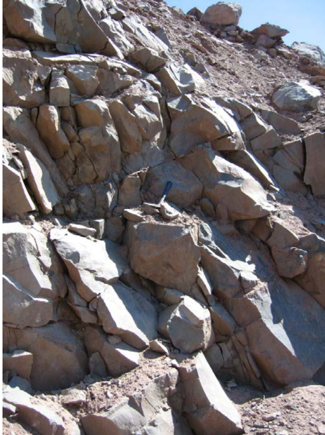
Figure 6. Highly jointed and fractured volcanic rocks of Quaternary age located on face of quarry cut slope proposed for expansion. Rock hammer visible at center for scale. (Photo by Will Arcand; dated August 2, 2006).
