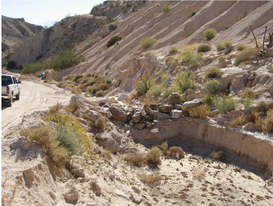
Figure 2. Rock check dam and sediment catchment basin placed at toe of gullied mine tailings slope. This structure was required to be redesigned in order to effectively control sediment eroding from the slope (Photo by Will Arcand; November 18, 2010).
