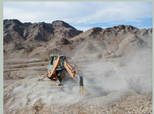
Backfill of the Golden Queen Mine in Imperial County during remediation.
