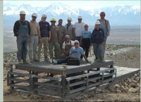
A completed bat cupola at the Southern Belle Mine in Inyo County. The cupola was constructed as part of an AMLU bat cupola and bat gate training class.
