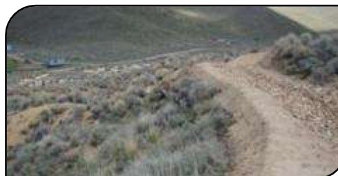
A lined diversion ditch (right) prevents runoff from eroding mine tailings (light colored soil on left).
