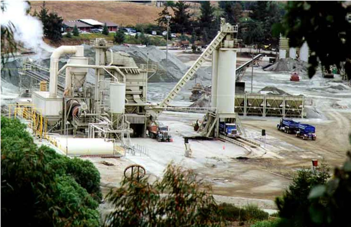
Granite Rock Company's fully automated 450-ton per hour asphalt batch plant located at the Arthur R. Wilson Quarry, San Benito County. A slat conveyor brings the asphalt to the load silo. The asphalt aggregate is Cretaceous hornblende gabbro mined from the Wilson Quarry, California's largest crushed rock mine. (Photo by Don Dupras, California Geological Survey)
